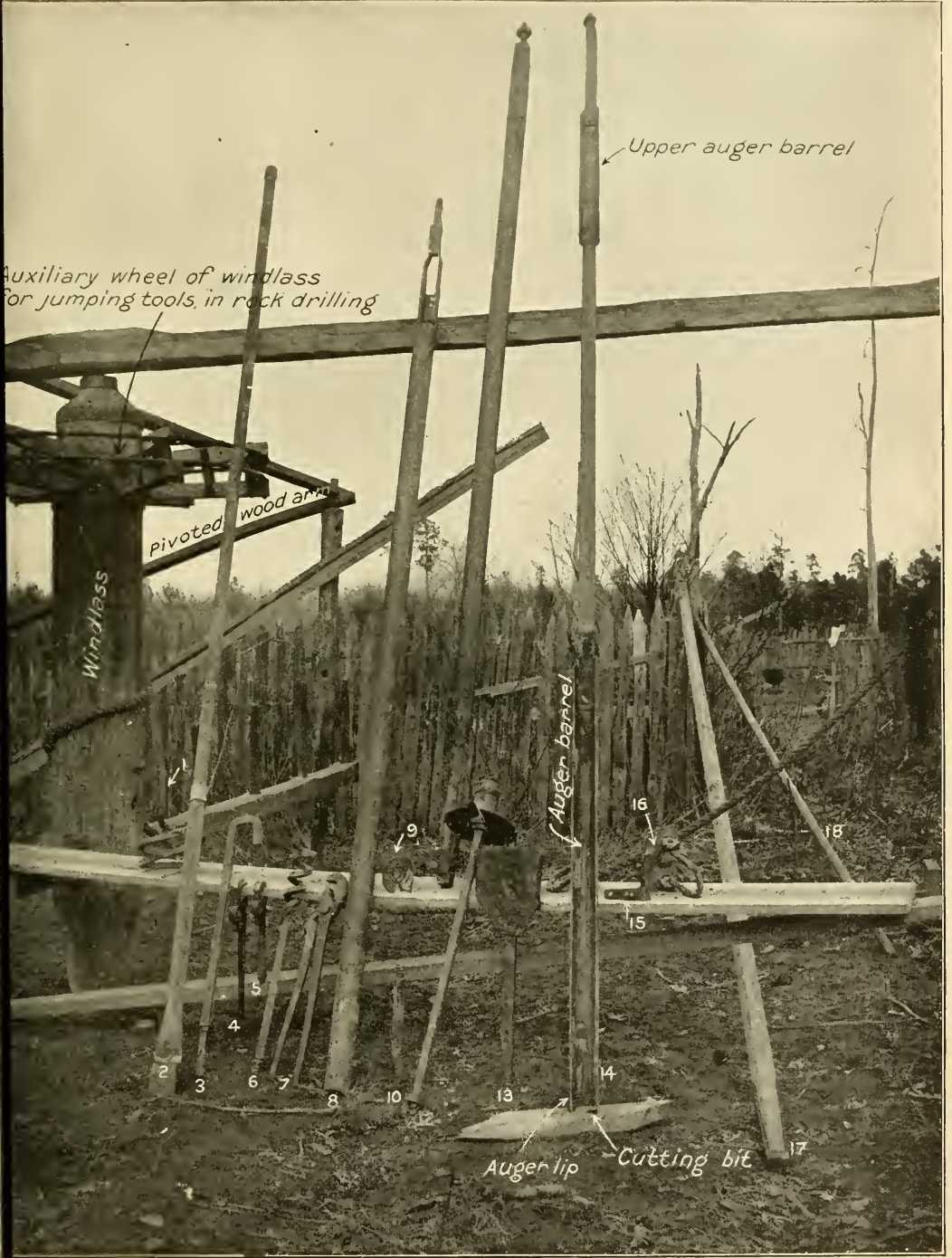
TOOLS OF AN ARKANSAS WELL-BORING OUTFIT.
