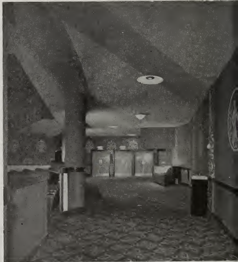
Continuous with the auditorium, foyer of the MacArthur theatre has been given a related treatment, with the plaster walls painted aqua blue as a ground for medallions and scrolls painted in white. Recessed ceiling luminaires provide illumination here, augmented by illuminated glass brick pylons at the aisle heads. The wainscot here, like that in the auditorium, also standee rail, are finished in leather-textured plastic.
