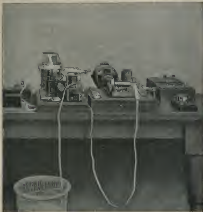
FIG. 1.—Complete receiving-printing apparatus, including receiving perforator with relay and printer.
