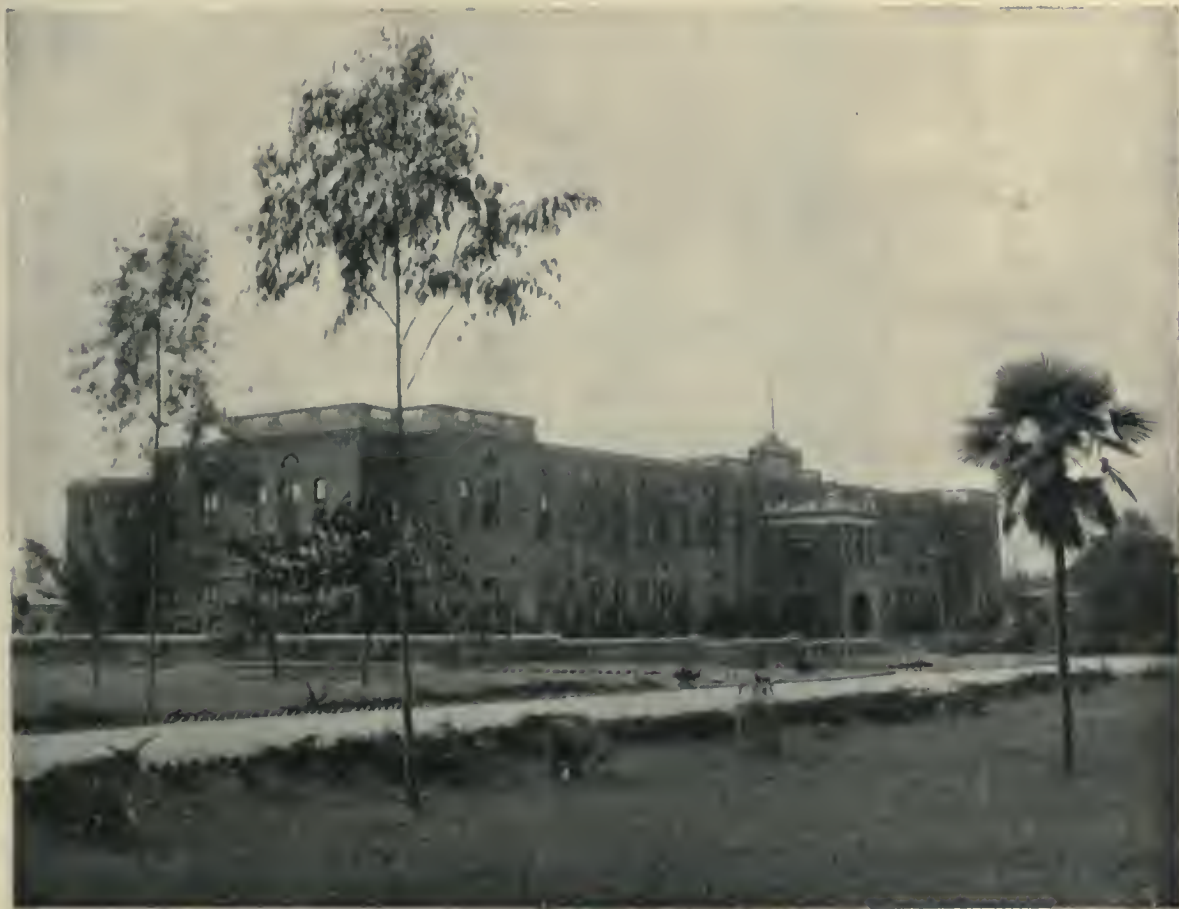
FIG. 1.—Main building of the Forest Research Institute, Dehra Dun. From "The Work of the Forest Department in India."
