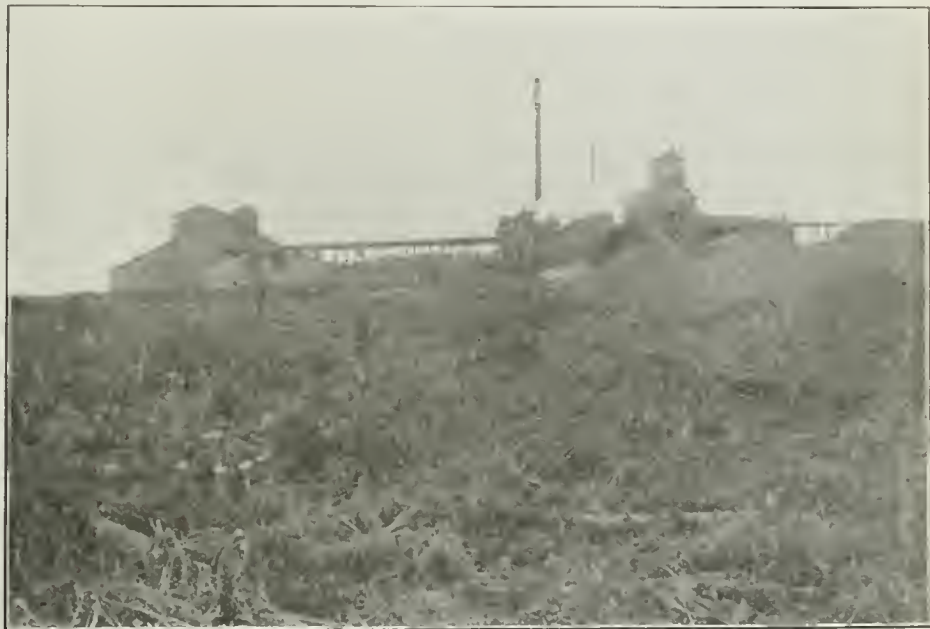
Massey Station copper mine, oil concentrator and mine looking west.
