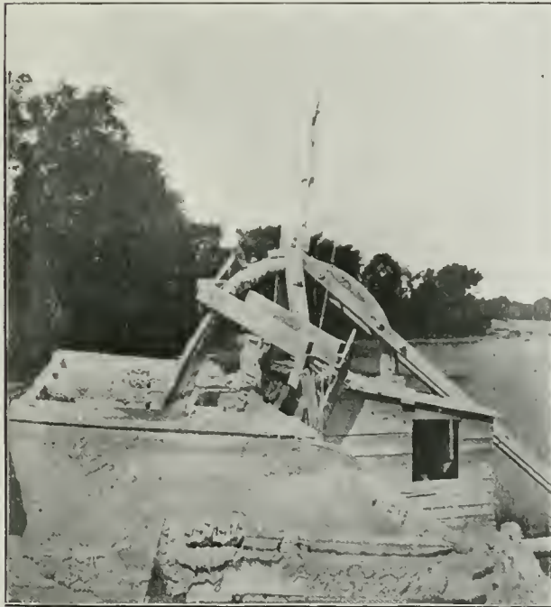
National Portland Cement Company. The Harris pneumatic system of pumping marl.
