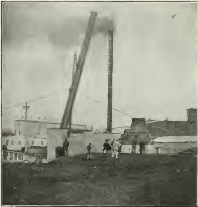
The Canadian Portland Cement Co., Marlbank plant. In the little “bottle” kiln shown in this picture was manufactured the first Portland cement made in Canada.
