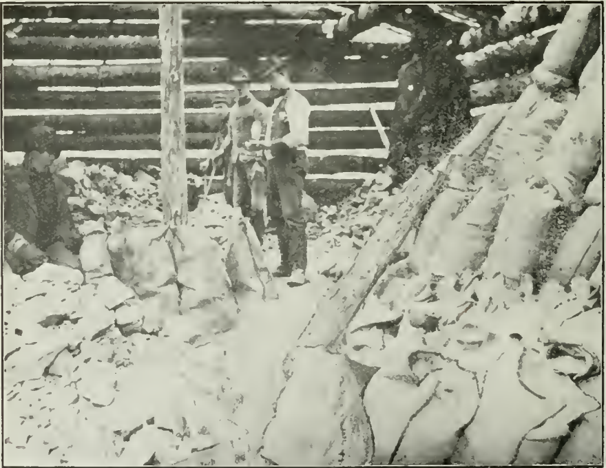
Fig. 23. Cobbing and sacking ore at the La Rose mine, November 1904.
