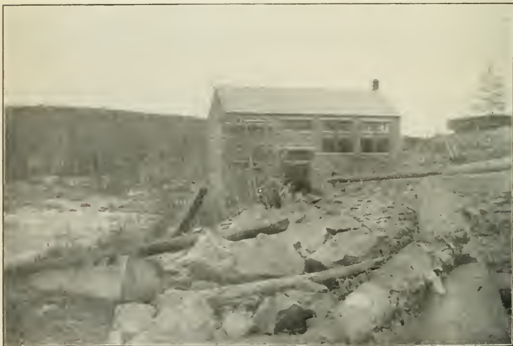
Power house of the Sudbury Power Company, McPherson falls, Vermilion river, Creighton township.
