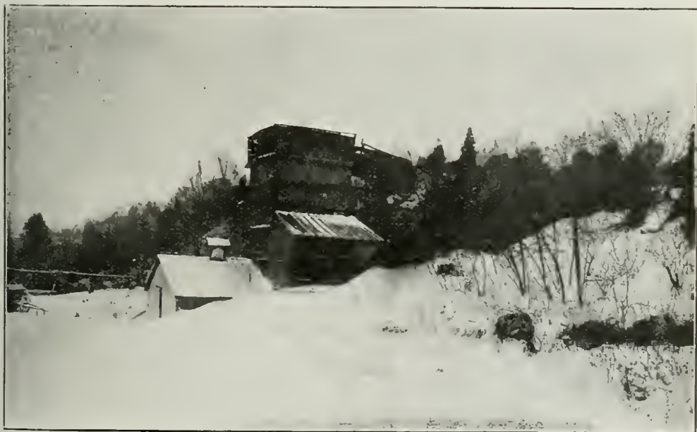
The Toronto Lime Co., Limehouse. View of kiln for making natural cement.
