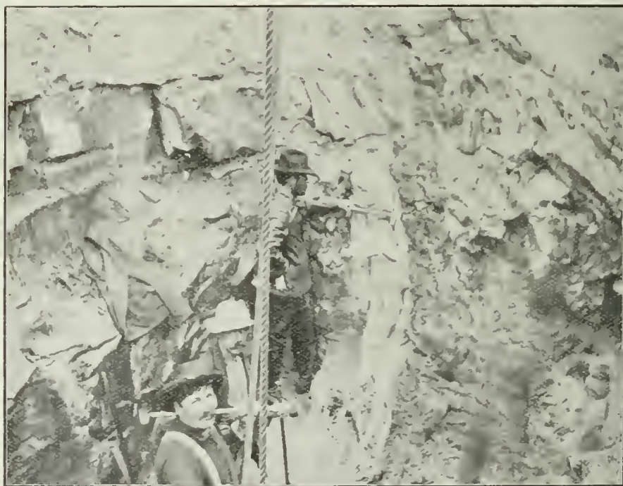
Fig. 7. Vein showing on the wall of a pit at the La Rose mine November, 1904. The width of the vein is equal to the space between the head of the hammer and the man's hand on the handle.
