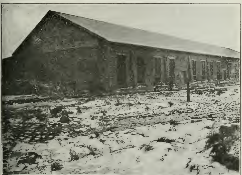
Superior Portland Cement Company, Orangeville. Main building.
