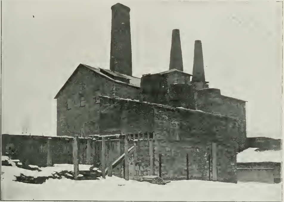
The Canadian Portland Cement Co., Strathcona. The rectangular stack to the left is that of two Dietsch kilns. The two to the right belong to two Alborg kilns. The three low kilns in the foreground are of the intermittent "bottle" type.
