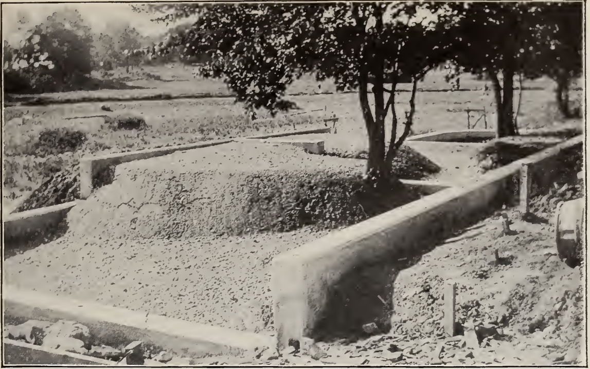
OTTER POOLS BEFORE ERECTION OF FENCES AND BEFORE TURNING ON WATER.
