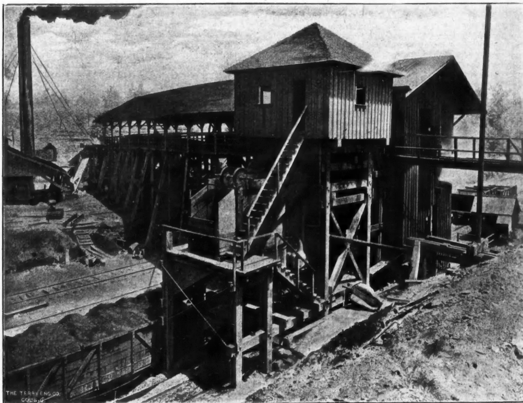
COAL WASHING PLANT AT NO. 2 SLOPE, TENNESSEE COAL, IRON AND RAILROAD COMPANY.
