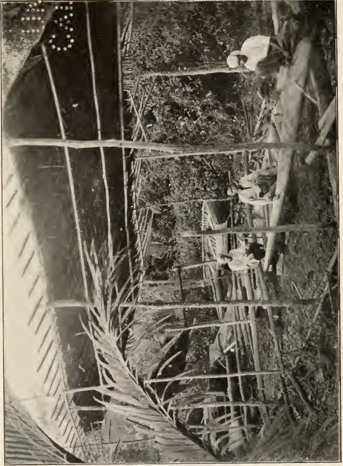
BOAT BUILDING—SPREADING THE BOTTOM.
