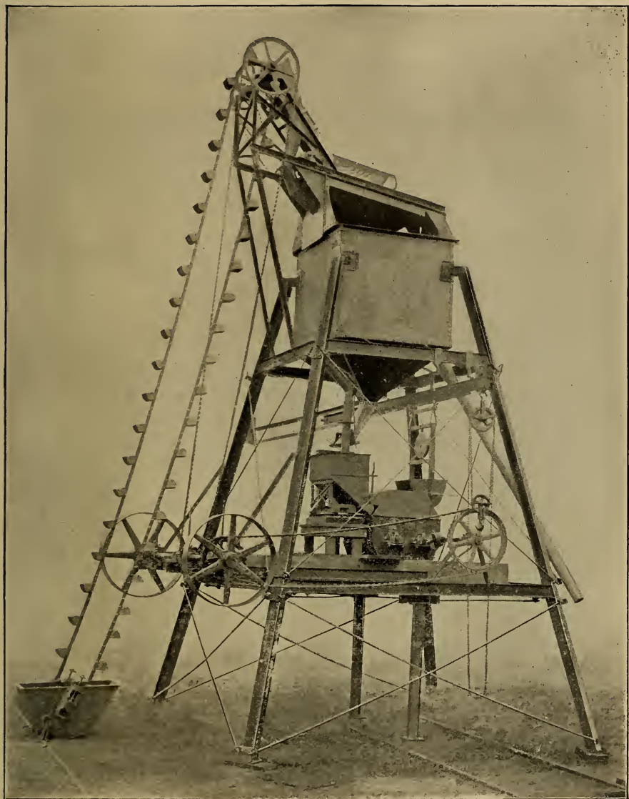
FIG. 14.—Semi-portable Mixing Platform.
