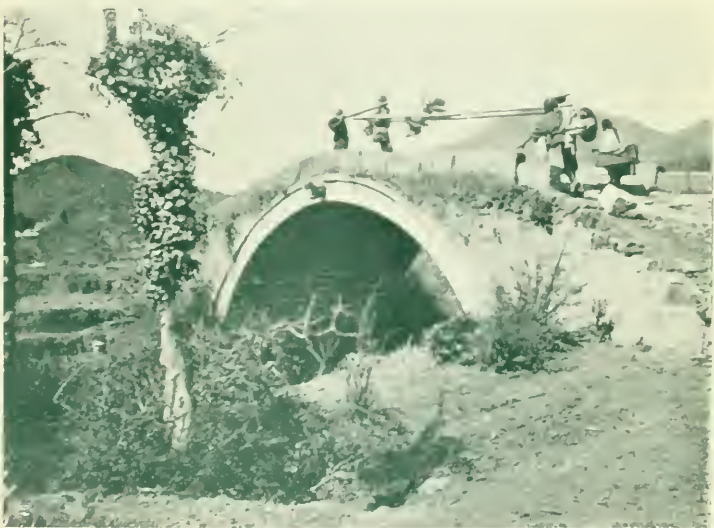
TWO STONE ARCH BRIDGES IN FAR WESTERN CHINA.
