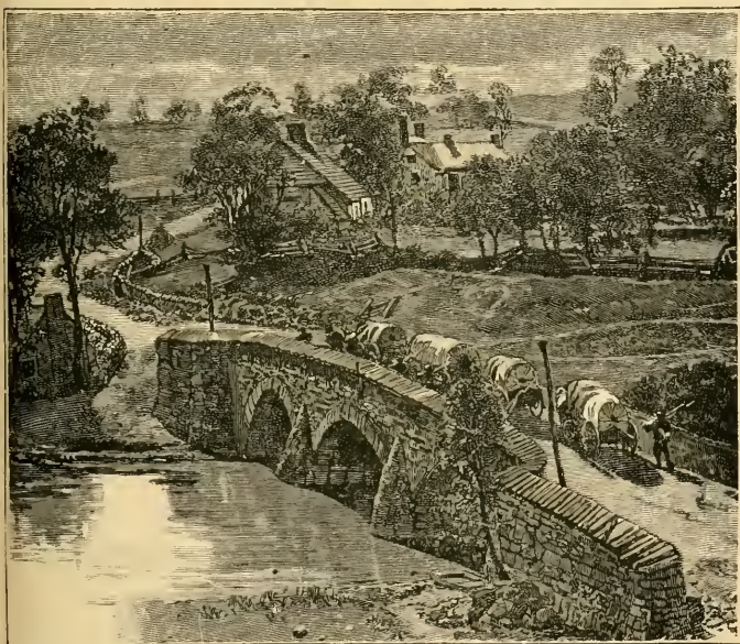
BRIDGE OVER THE ANTIETAM. 1
