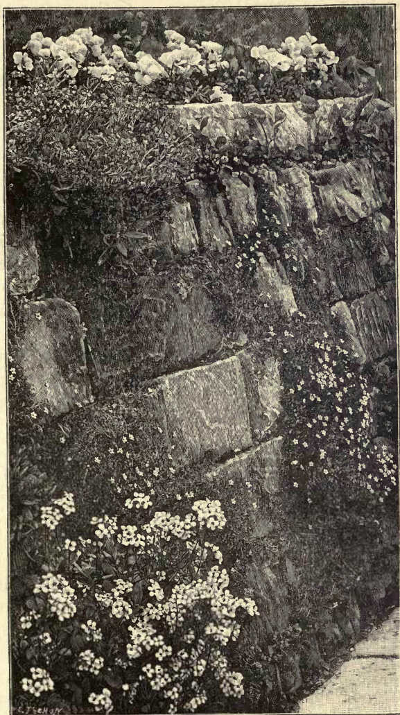
Sloping wall of local sandstone, supporting banks on each side of path, rock plants placed between each line of stones as wall was built. (Engraved from a photograph taken in my garden, by G. A. Champion.)
