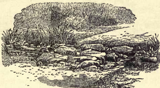
Stepping-Stone Bridge, with Water-Lilies and Water Plants.
