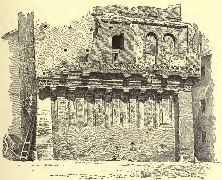
The House of Crescentius.
