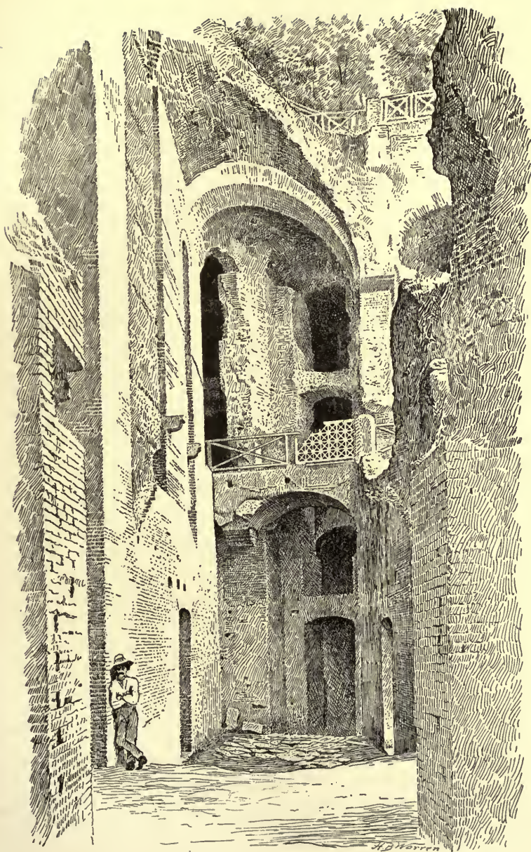
SUBSTRUCTIONS OF THE PALACE OF CALIGULA.
