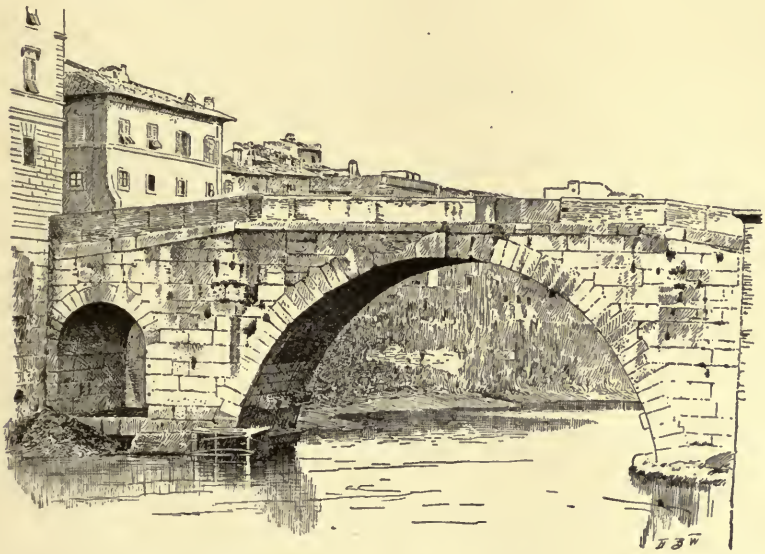
Bridge built by Lucius Cestius.
