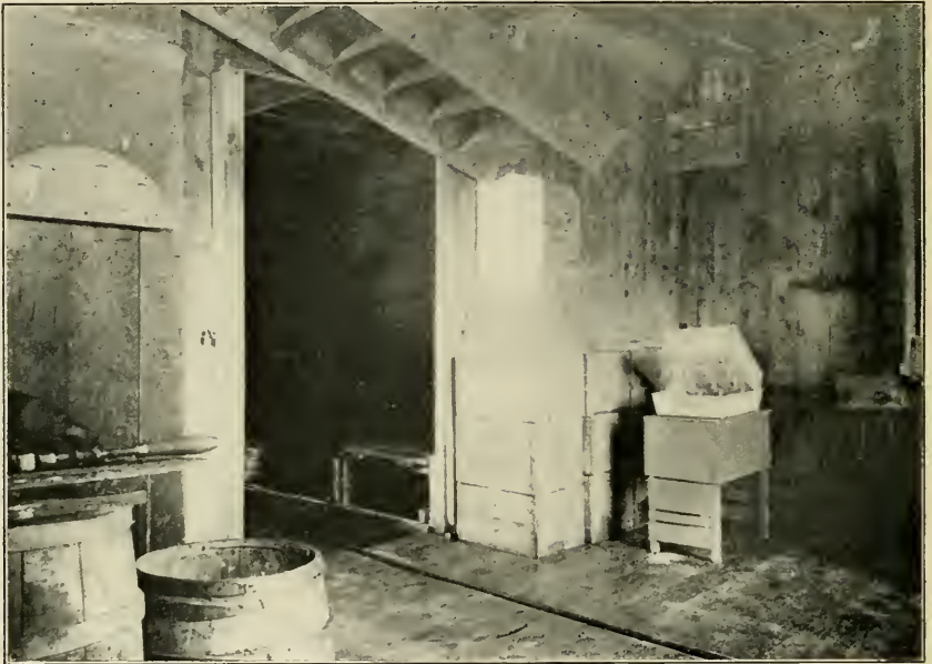
NARROW CENTER FLOOR GUTTER.
