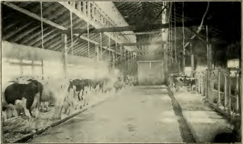
INTERIOR OF COW STABLE, SHOWING CLEAR STORY METHOD OF CONSTRUCTION.
