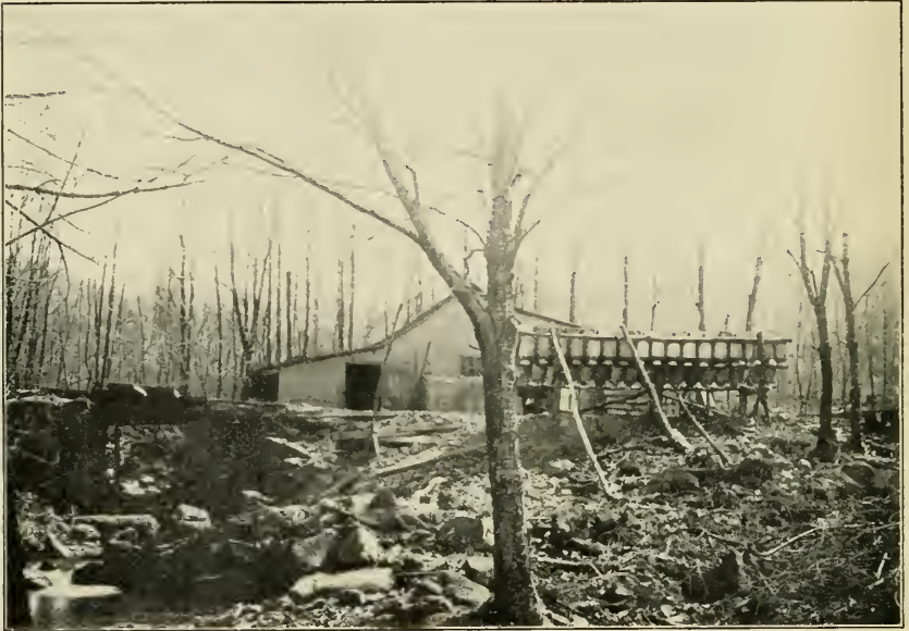
CREAMERY WITHOUT PROPER LIGHT, VENTILATION OR EQUIPMENT.
