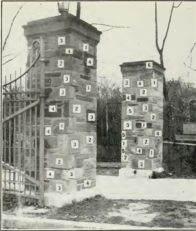
1. THE PILLARS TO THE RIGHT OF THE HARVARD STREET ENTRANCE TO THE ZOO. WITH BUILDING BLOCKS NUMBERED AS EXPLAINED IN TEXT.
