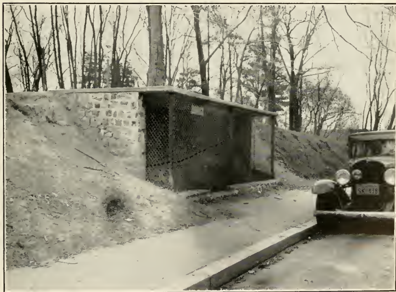
2. SHELTER CONTAINING OVERTHRUST FAULT EXHIBIT ALONG ADAMS MILL ROAD NEAR ZOO GATE. FAULT INDICATED BY DOTTED LINE.
