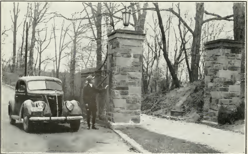
2. STONE PILLARS ON RIGHT SIDE OF ADAMS MILL ROAD ENTRANCE TO ZOO, WITH DONALD F. MCHENRY OF NATIONAL PARK SERVICE.
