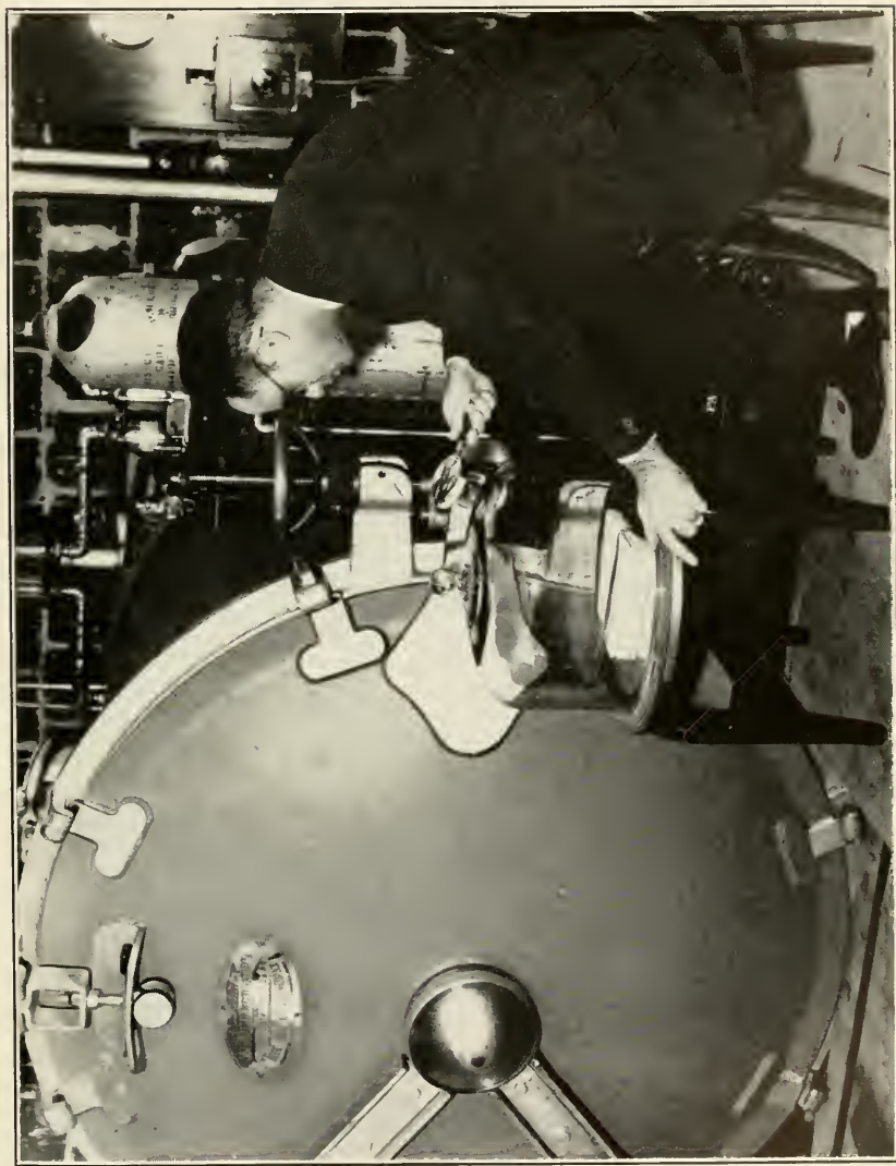
VIEW OF CYLINDRICAL STEEL VACUUM FUMIGATOR INSTALLED IN THE HUNTINGTON LIBRARY.
