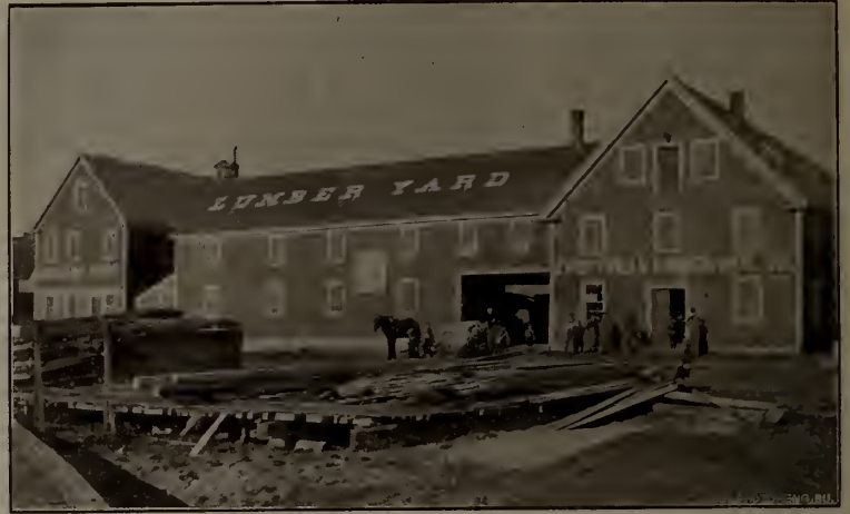
KEMPTVILLE LUMBER MFG. CO.'S FACTORY, YARMOUTH, N. S.
