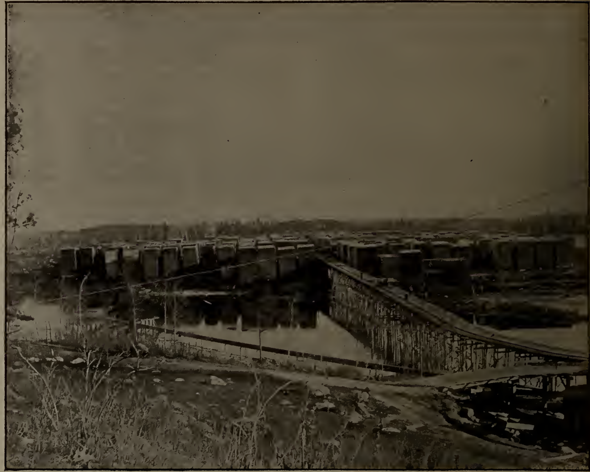
PILING GROUND OF THE ONTARIO AND WESTERN LUMBER CO. AT RAT PORTAGE.
