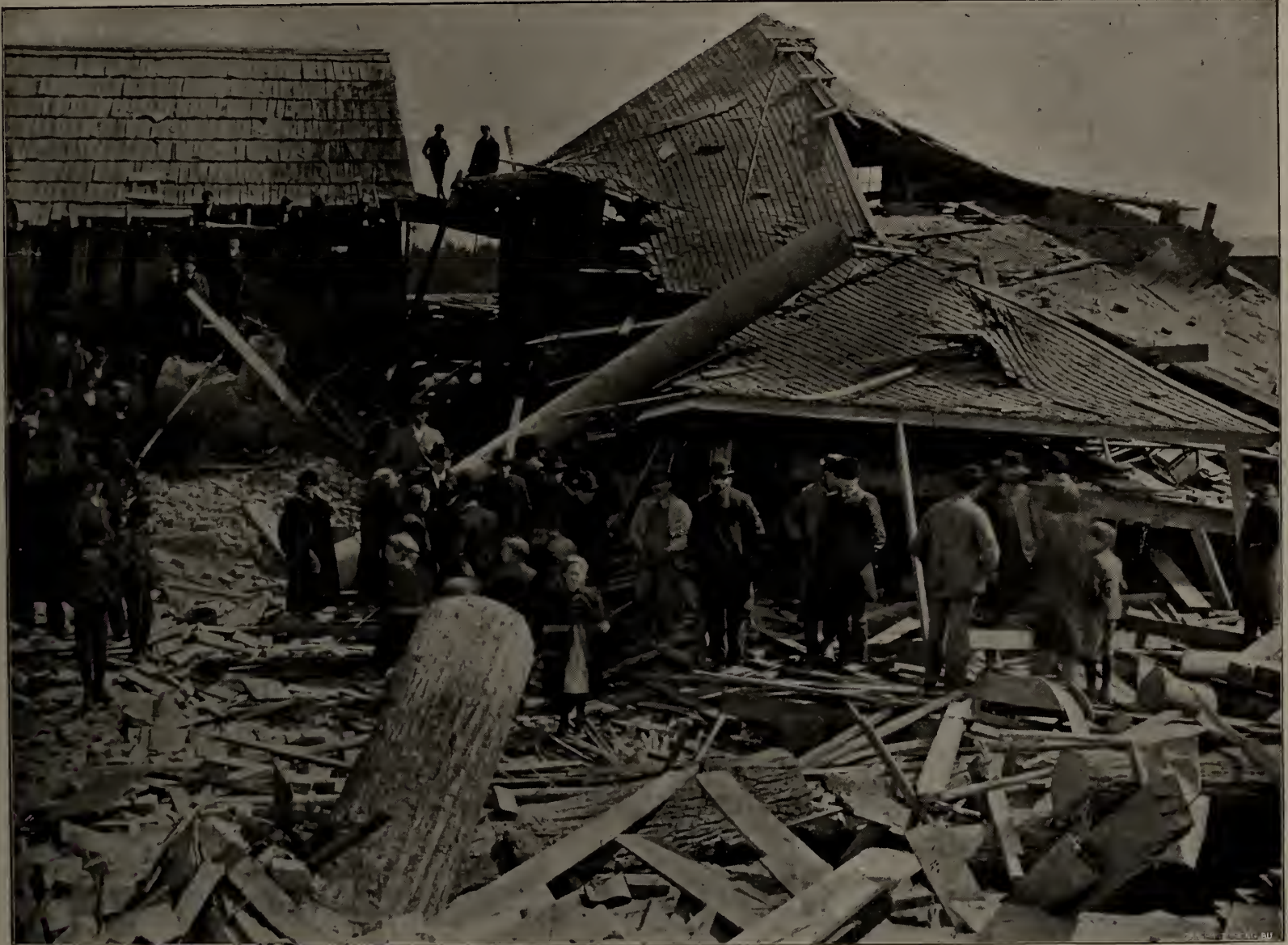
BOILER EXPLOSION AT RIDGETOWN, ONT.
