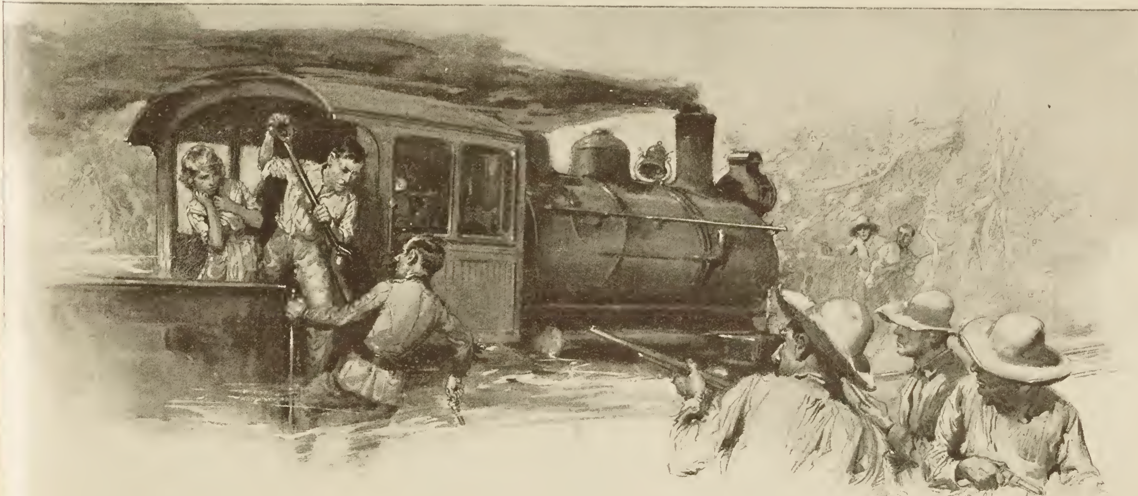
MORE MEN WERE AHEAD, GROUPED AT THE BASES OF THE ROCK SPURS THAT BUTTRESSED THE CUTTING
