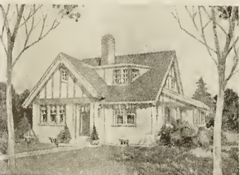
Half Timber Treatment
