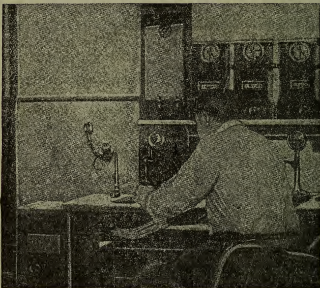
Train Dispatcher's Desk, Showing Selective Signaling Devices and Telephone Sets.
