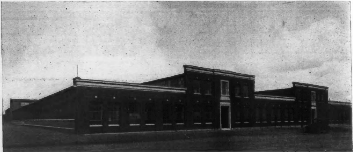
Exterior of The Reg. N. Boxer Co., Ltd., New Toronto; Designed, Built and Equipped by The Austin Company
