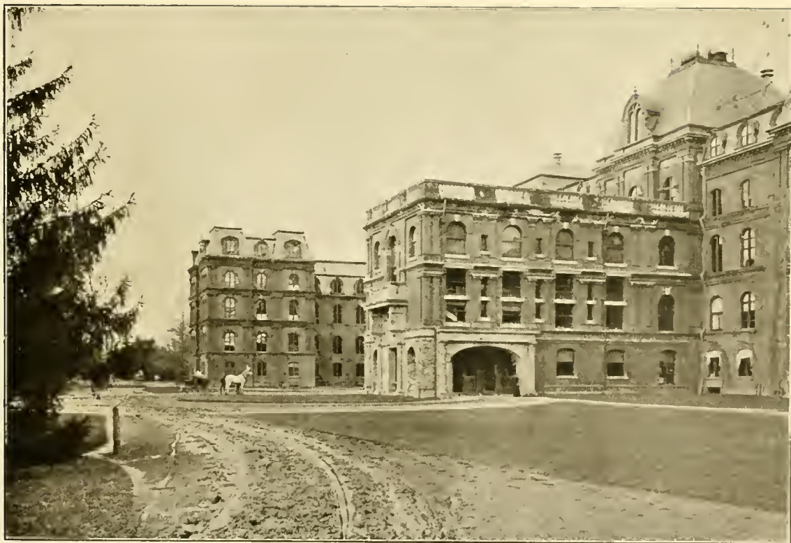
LIBRARY AND MAIN BUILDING, VASSAR COLLEGE.
