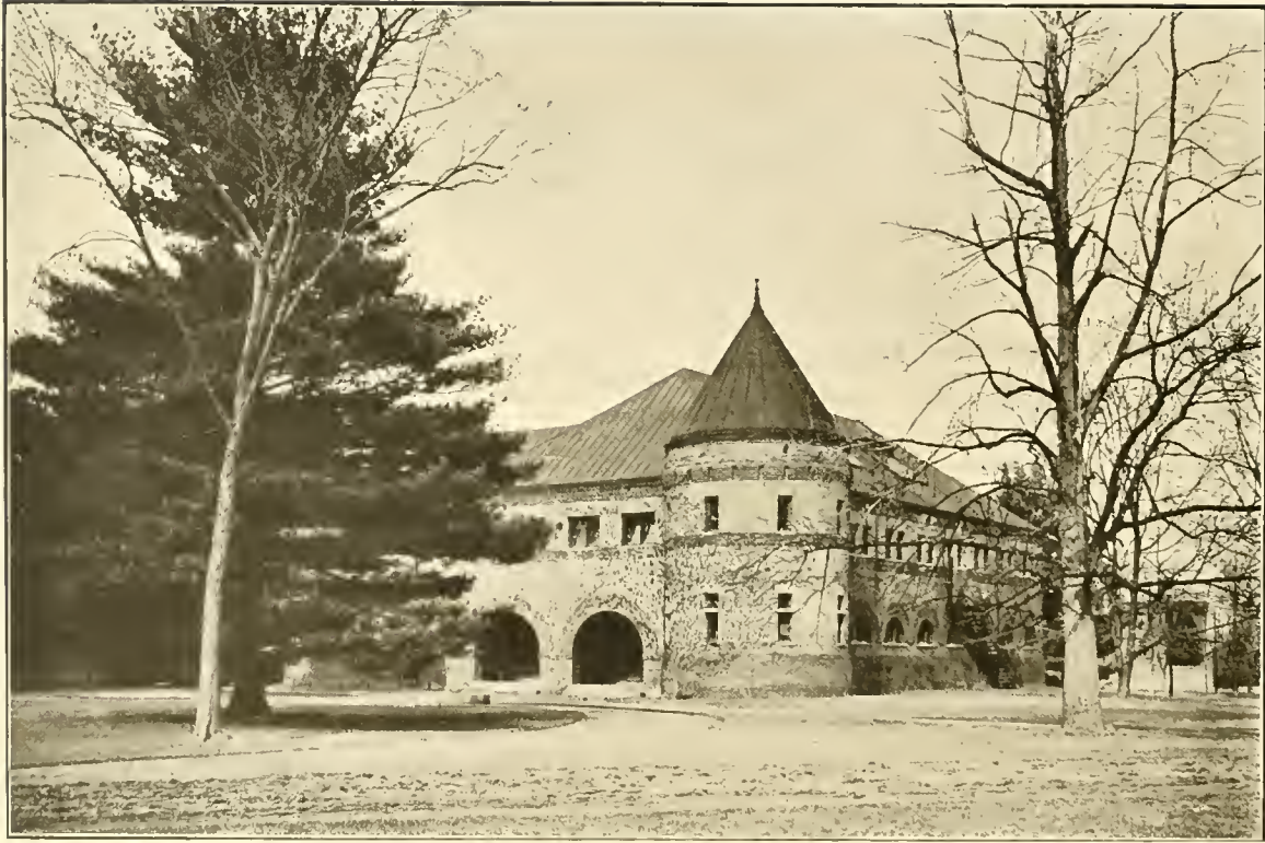
THE GYMNASIUM, VASSAR COLLEGE.
