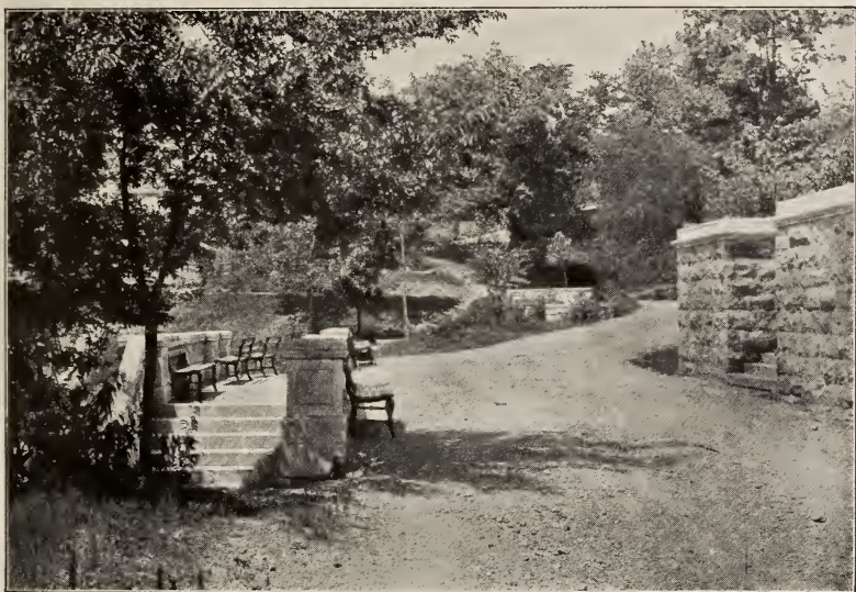
ON HOT SPRINGS MOUNTAIN, HOT SPRINGS OF ARKANSAS
