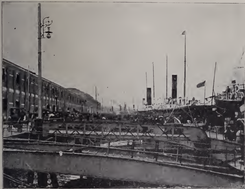
WHARF AND STOREHOUSES, SHANGHAI.
