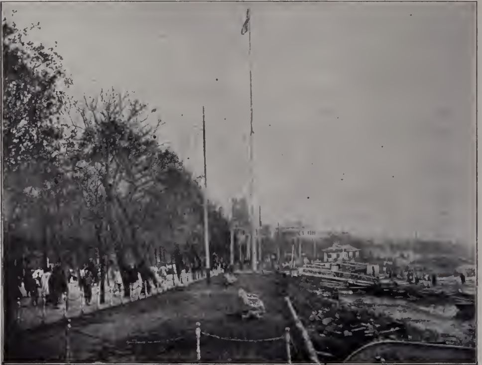
ROAD BY THE SIDE OF WANGPOO RIVER, SHANGHAI.
