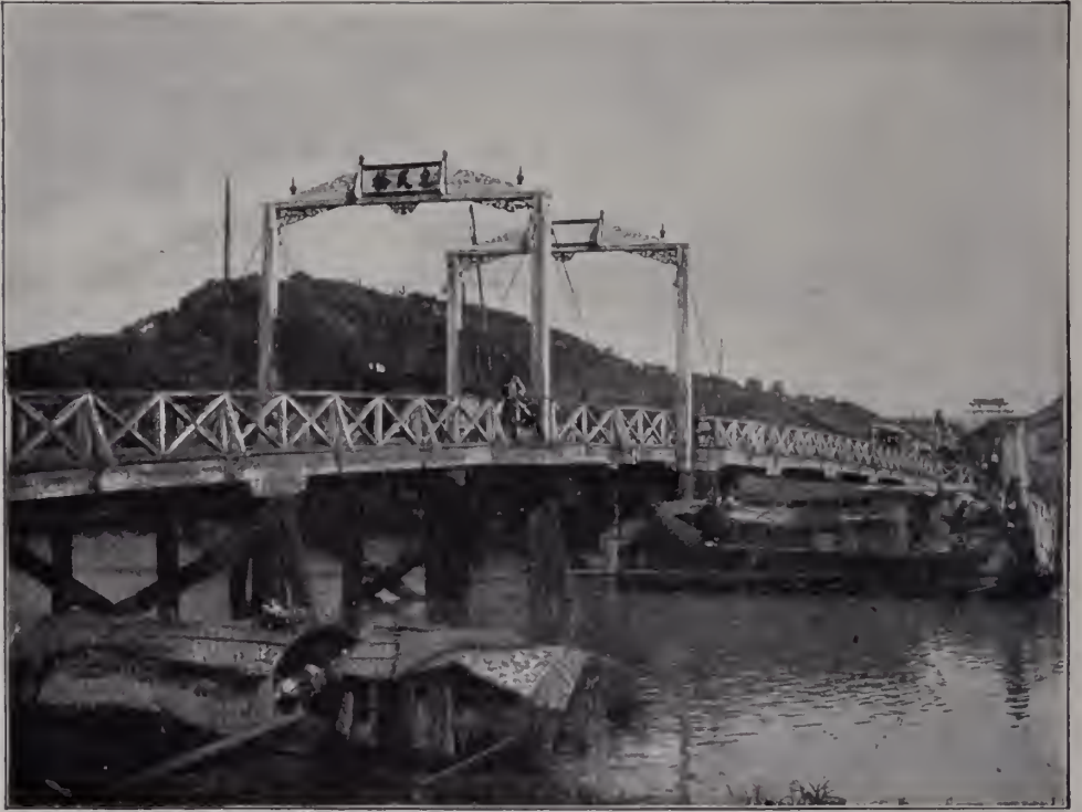
DRAWBRIDGE CONNECTING WHARF AND CITY, NANKIN.
