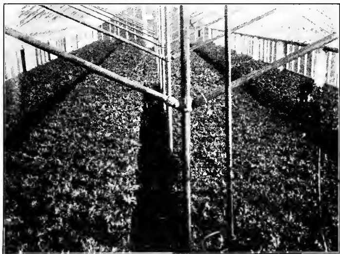
FIG. 28. A COMMON FORM OF GREENHOUSE BRACING
