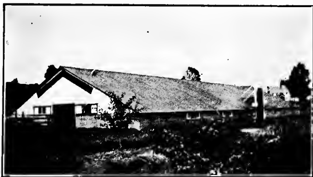
FIG. 80. CELERY STORAGE HOUSE
