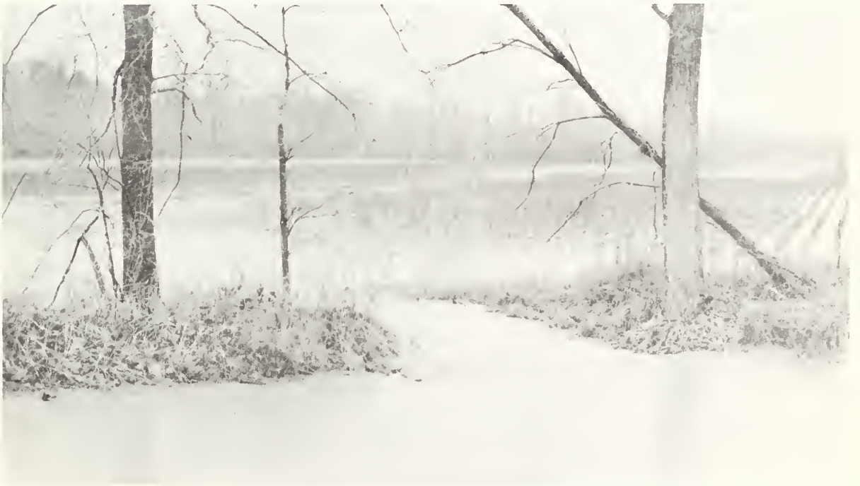
Floodwaters on Roland Branch spilling over levee. This levee had to be rebuilt several times in the past few years.
