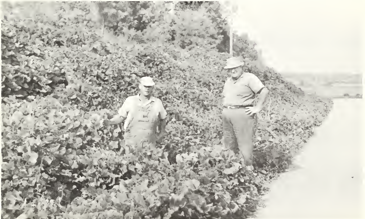
Similar roadbank as shown above after being stabilized with kudzu crowns.
