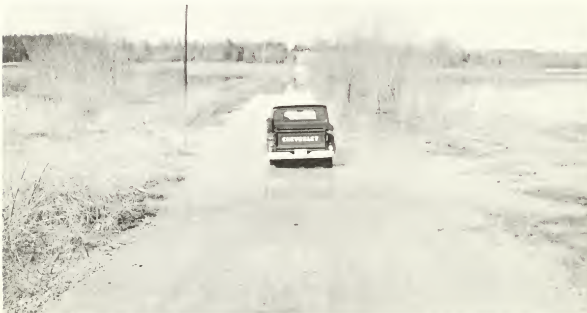
This picture shows a county road in Lower Cypress beginning to flood. Frequently, during larger floods, school children are transported by boat or horseback across this section.
