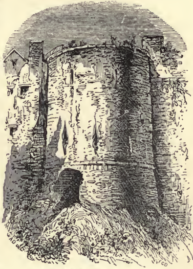
GARTER TOWER, FROM THAMES STREET
