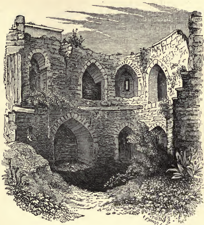
INTERIOR OF THE GARTER TOWER.
