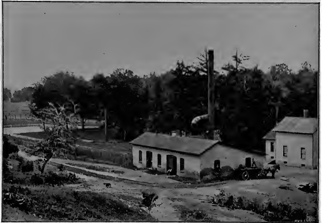
THE CITY WATER WORKS.
