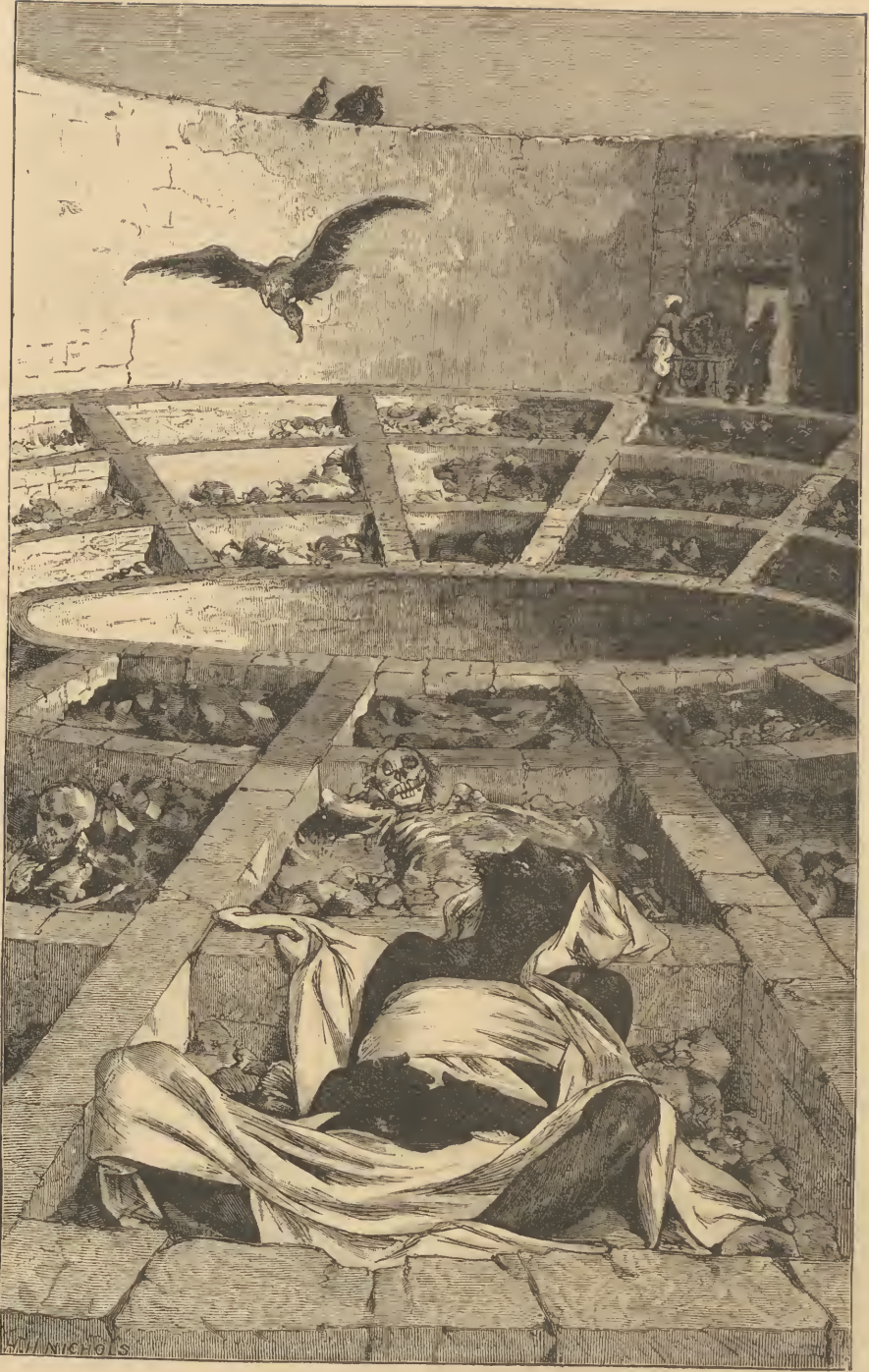
FIG. 3.—Parsee Towers of Silence (interior).
