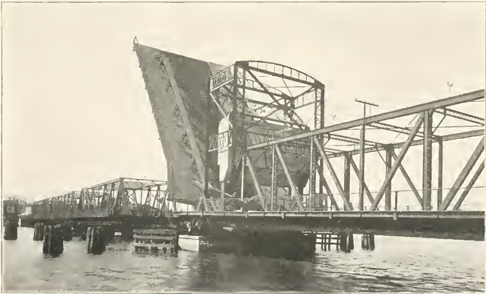
BASCULE BRIDGE, AT WALNUT STREET, GREEN BAY
