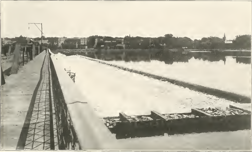
BRIDGE AND DAM, DE PERE
