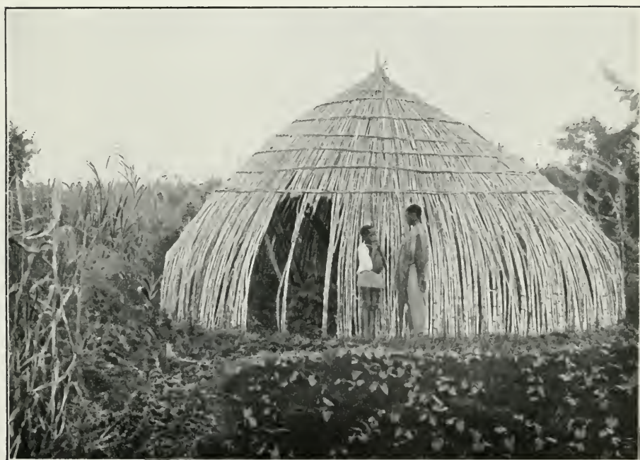
FRAMEWORK OF A WAHAIA HUT: BUKOBA DISTRICT
