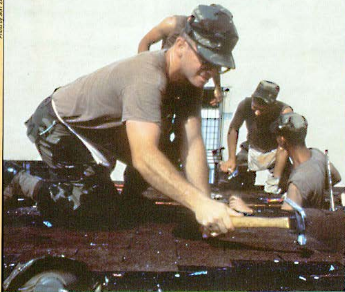
SGT Scott Anderson, 10th Mountain Div (L), Ft. Drum, NY, hammers shingles on a roof top at a local resident's home in Homestead AFB, FL as part of the Hurricane Andrew relief mission.
