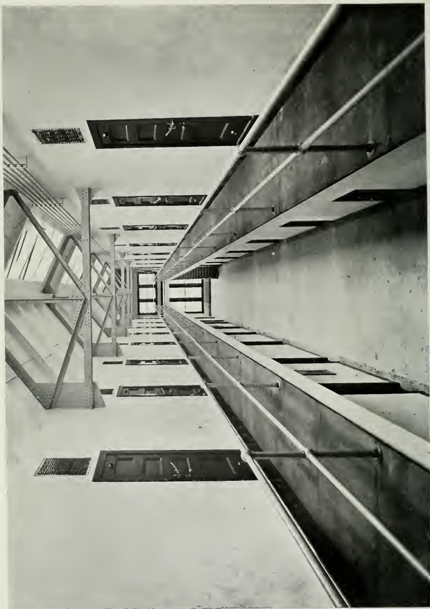
SOUTH SECTION OF WEST FAÇADE. Gallery showing fire-proof rooms for study and storage collections
