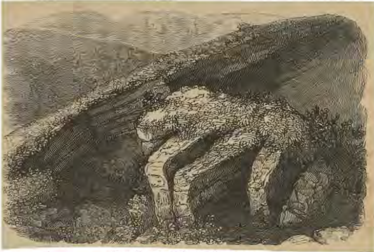
THE PALMER'S CAIEN LANDSLIP.
