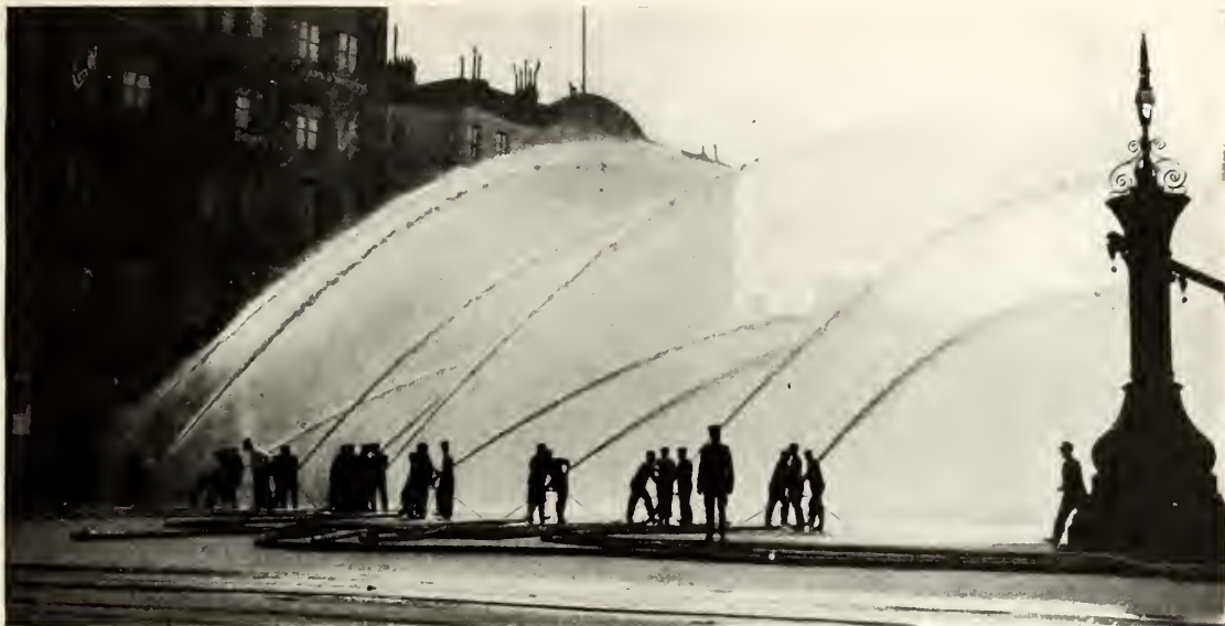
STARTING THE STREAMS FOR A HIGH-PRESSURE TEST IN UNION SQUARE.
