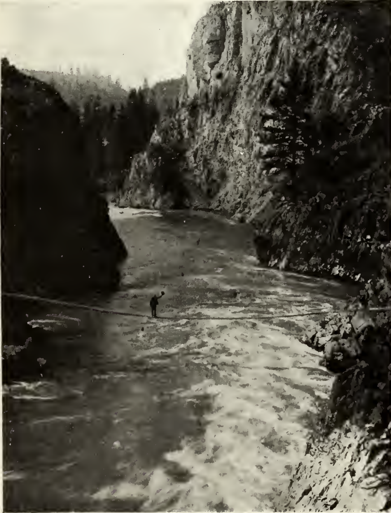
A CABLE BRIDGE SPANNING SPOKANE RIVER.
