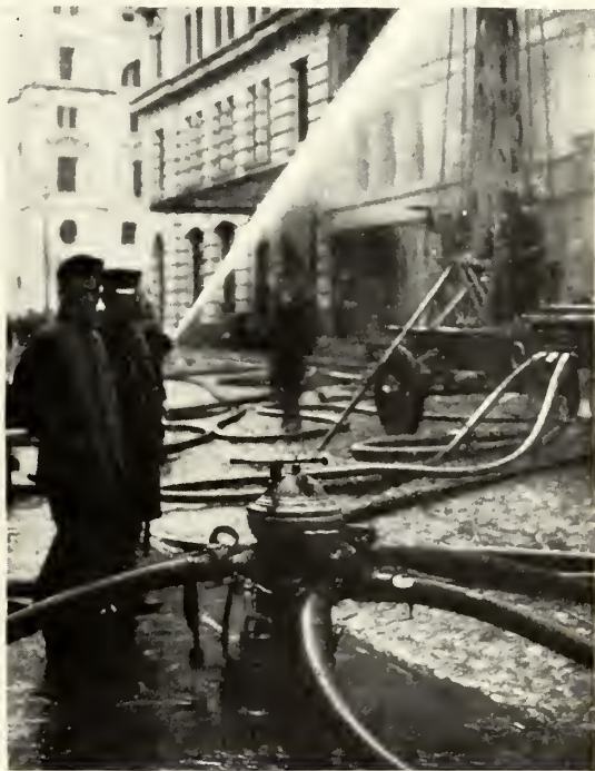
A HIGH-PRESSURE HYDRANT IN SERVICE, WITH AN ENGINEER (AT THE LEFT) IN CHARGE.
