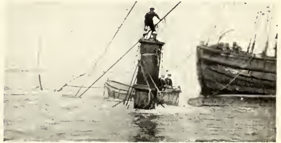
AN AIR-LOCK LEADING DOWN INTO THE SUBMERGED YANKEE .
