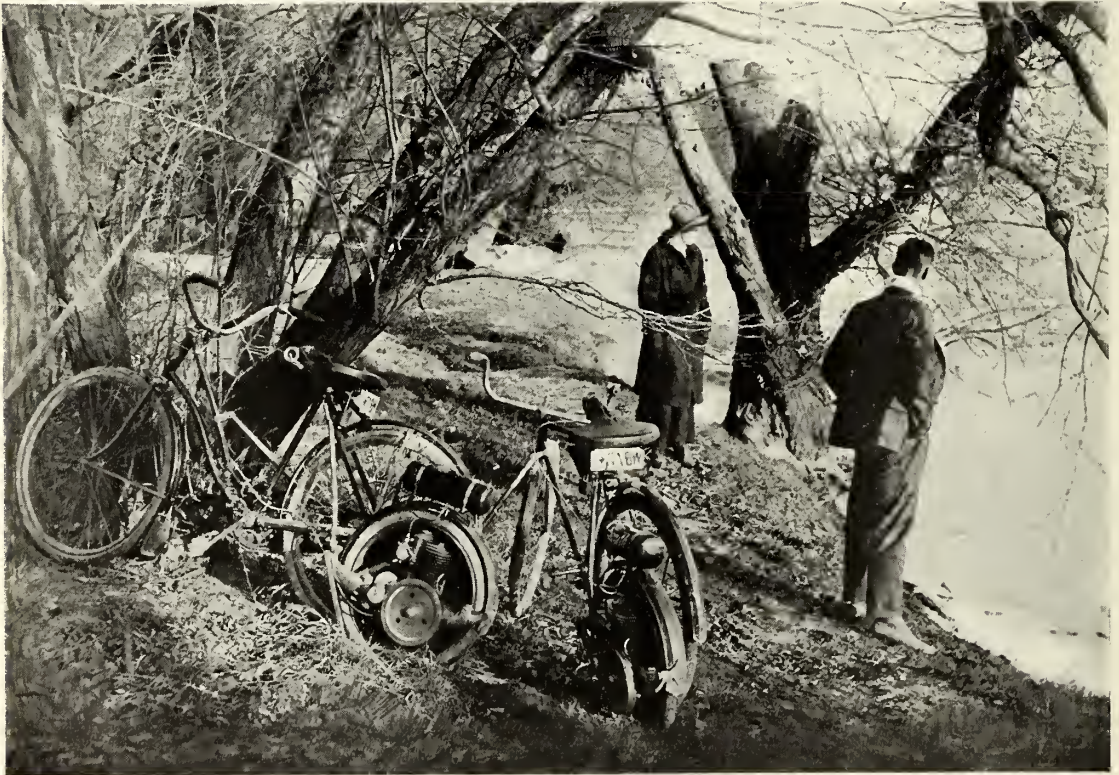
THE MOTOR-WHEEL—THE NEW ATTACHMENT FOR BICYCLES.
