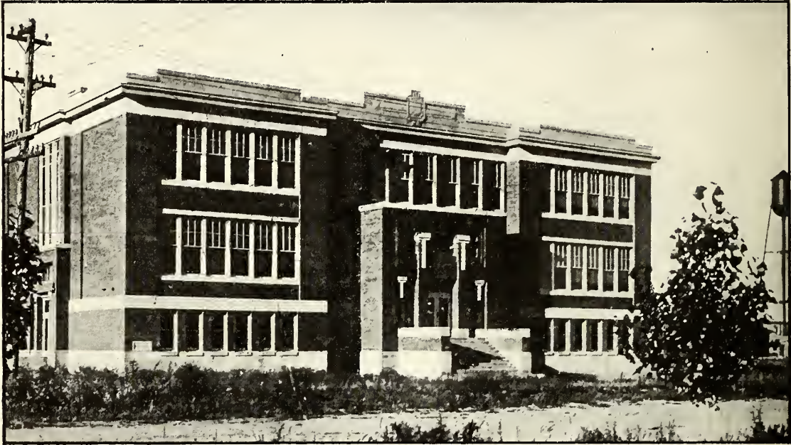
THE HIGH SCHOOL BUILDING AT RUPERT, IDAHO.
