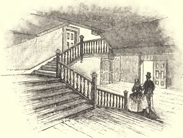
STAIRCASE IN ROBINSON'S HOUSE
