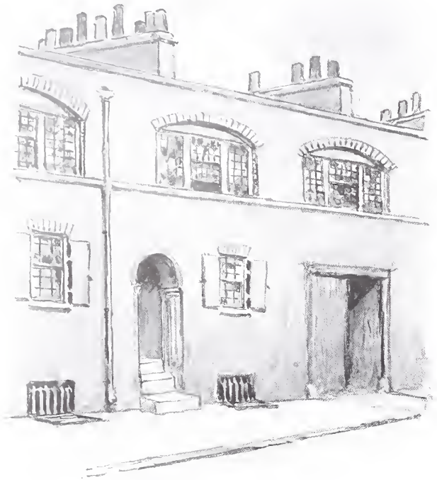
Weavers' Houses, Menotti Street, Bethnal Green. Showing large windows of workshops on top floor.
