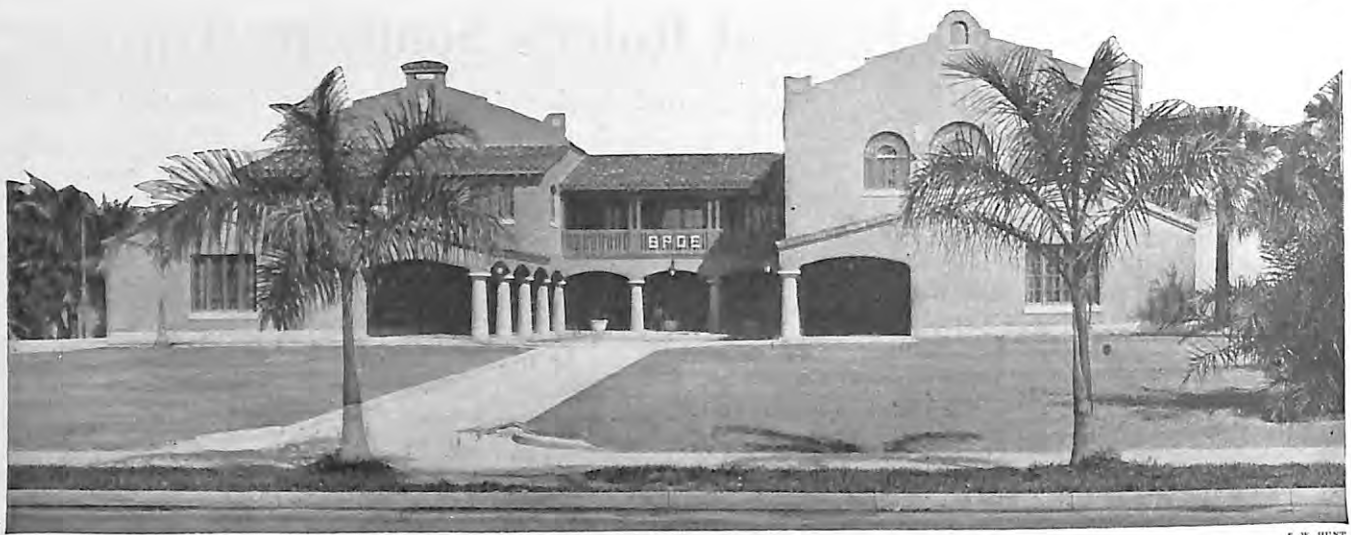
The magnificent new Home owned by Fort Myers, Fla., Lodge, No. 1288, characteristic of the fine Elks' buildings in Florida
