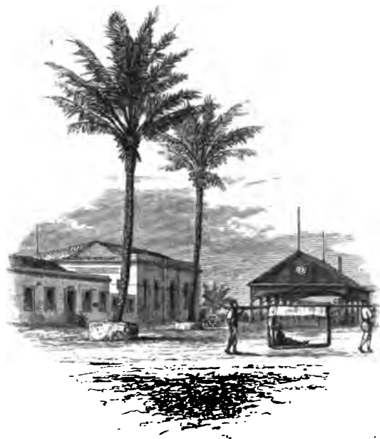
CUSTOM-HOUSE AT BENQUELLA.
