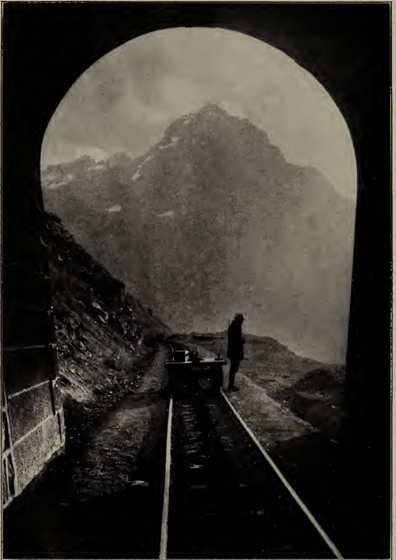
Most of the steepest grades on the Transandine Railway are on the Chilean side. Corkscrew tunnels like those of the Gothard route were too expensive, so the height is conquered by a rack and pinion system.
