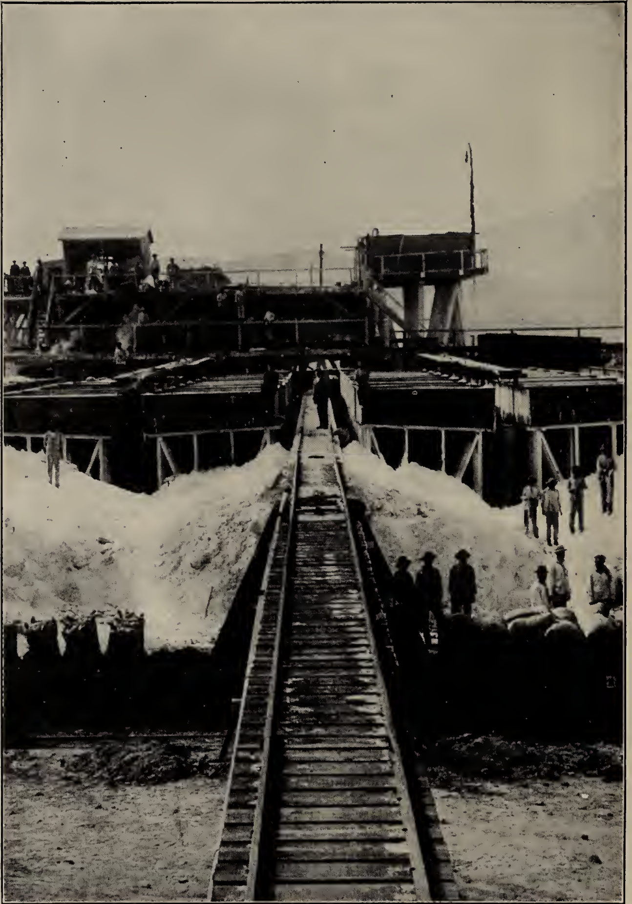
Nitrate is refined by melting the crude rock and then allowing the salt to settle in huge vats. As the water is drawn off, the snow-white chemical is left to dry.
