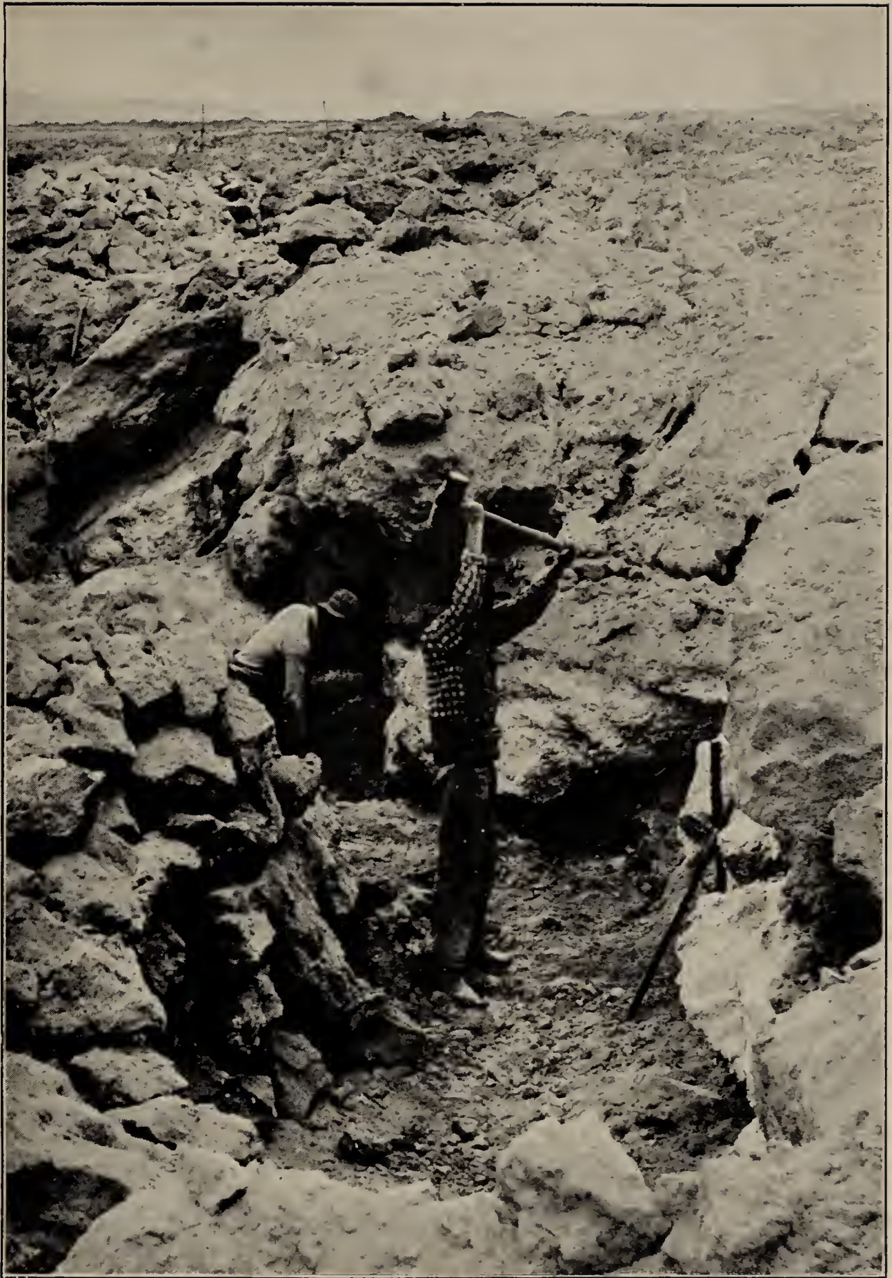
The nitrate deposits lie about twenty feet below the surface, and are mined by boring a hole into the ground and inserting a charge of dynamite. After blasting the salt rock is dug out with crowbars and picks.
