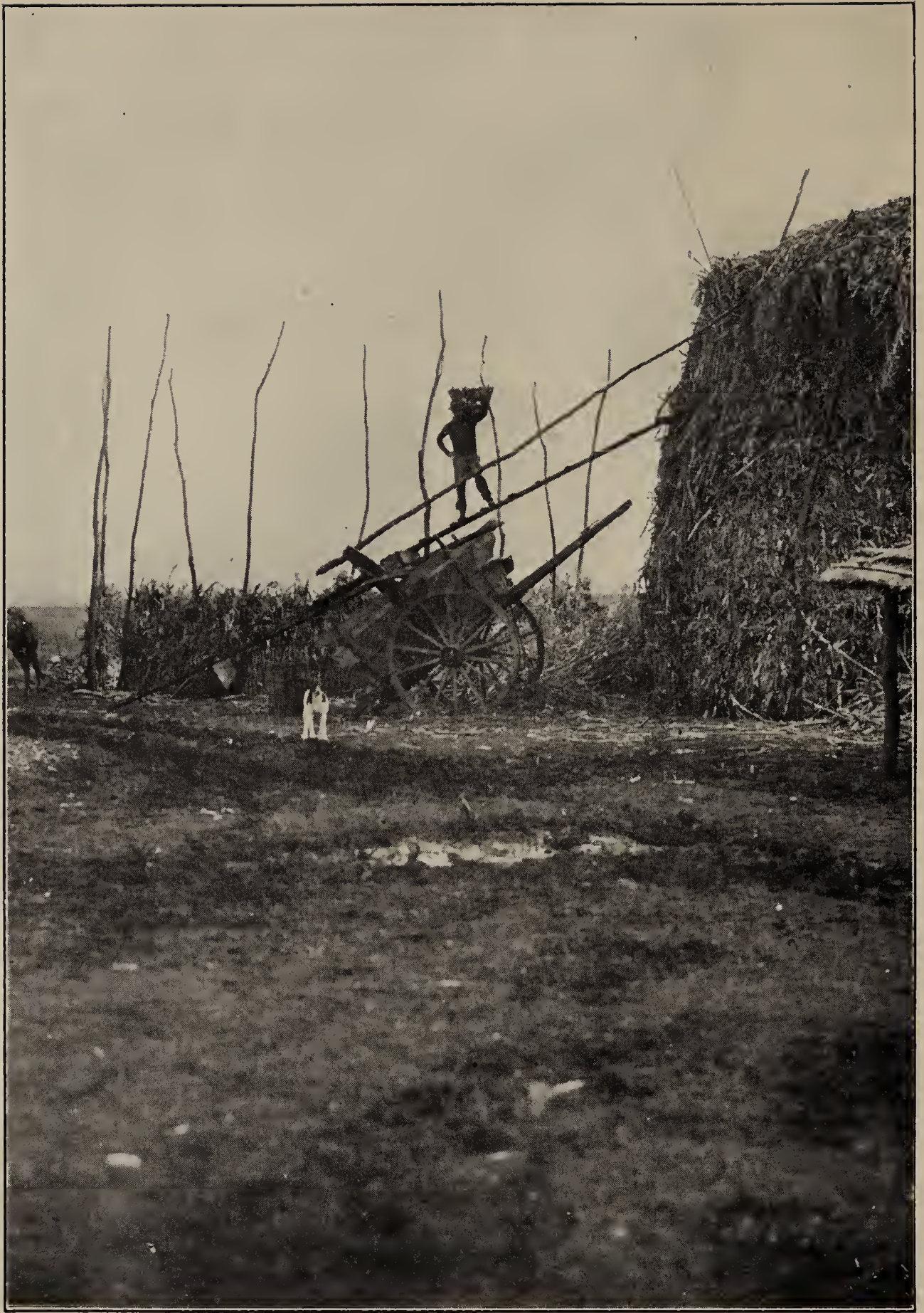
The Argentine "troje," or corn crib, is made of corn stalks so woven around a framework of poles as to protect the grain stored inside. Argentina is the world's chief corn exporter.
