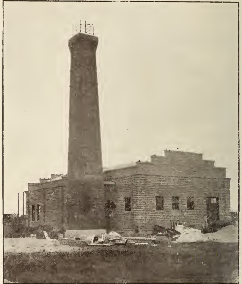
Power House of the Saskatoon Public Works, Electric Light Plant and Water Works Pumping Station.
