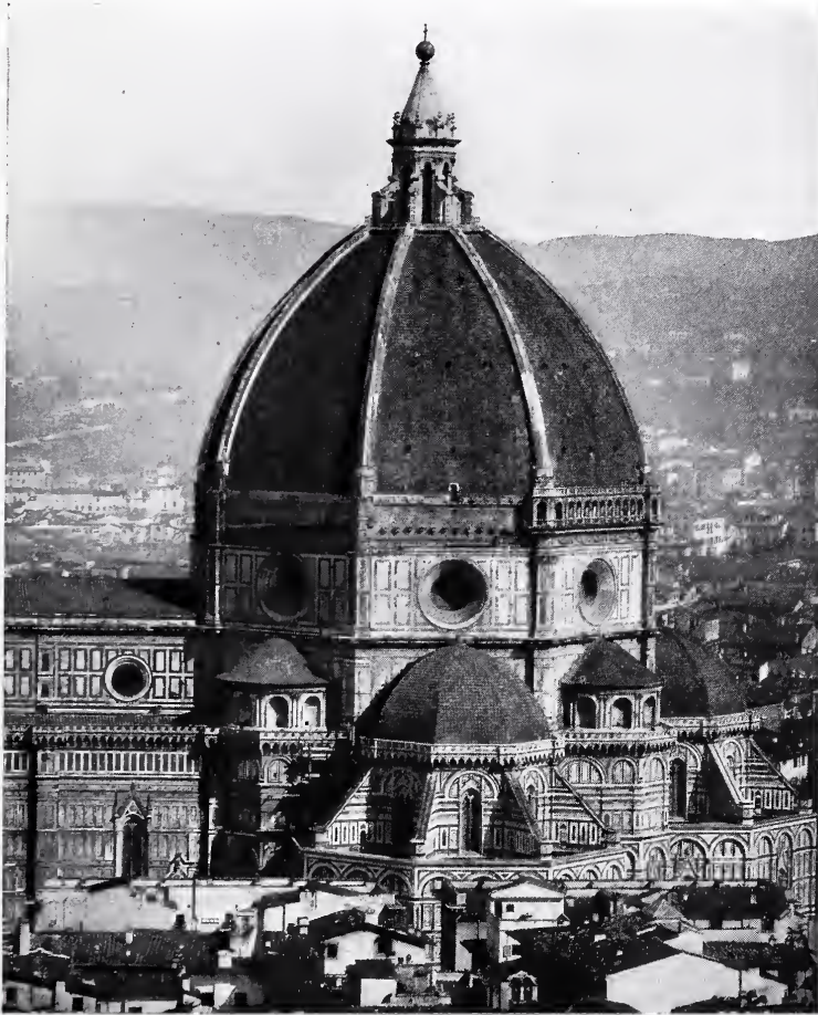
DOMES OF CATHEDRAL OF FLORENCE. DESIGN EXPRESSES STRUCTURAL SYSTEM; INVISIBLE STRAINS RESISTED BY CONCEALED BELTS.
