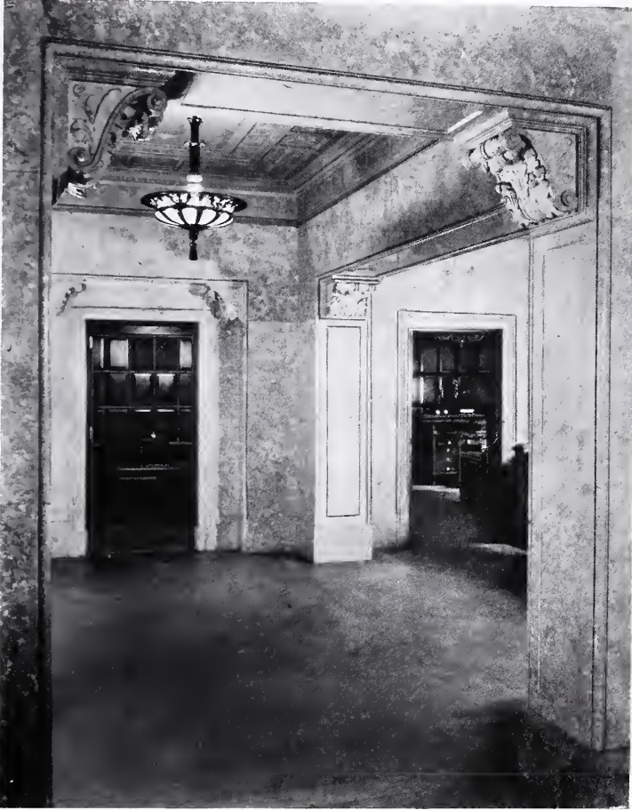
LOBBY OF PRESIDENT'S SUITE—GUARDIAN SAVINGS AND TRUST COMPANY'S BUILDING, CLEVELAND, OHIO. Walker & Weeks, Architects.
