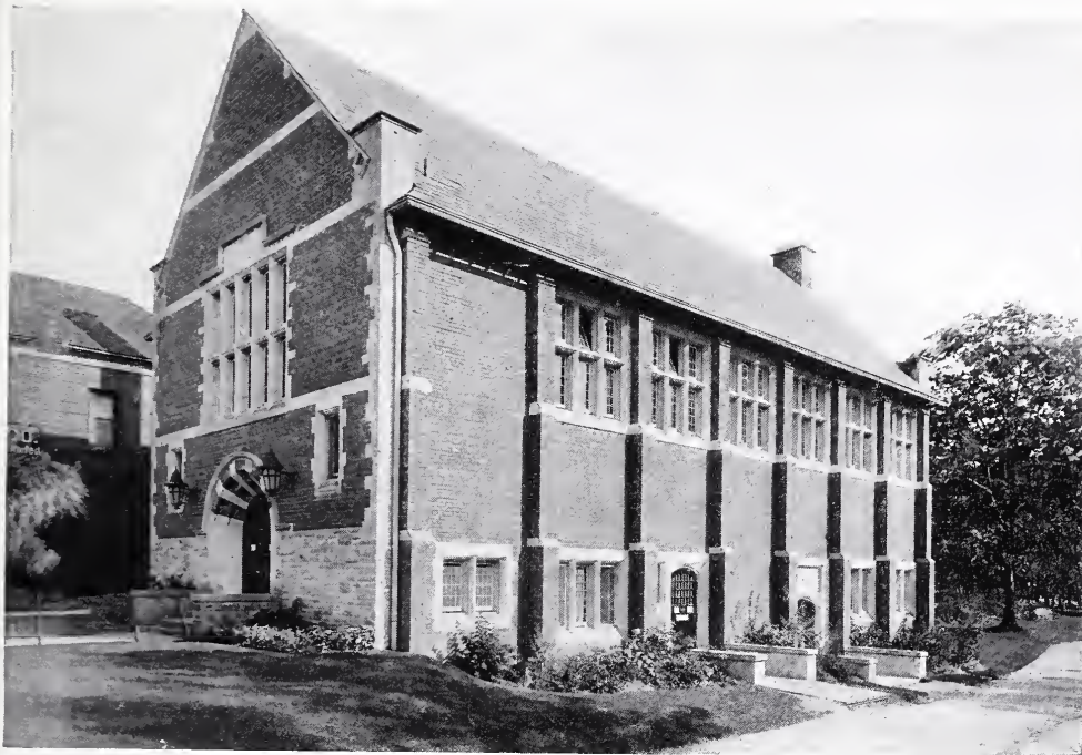
WYCHWOOD BRANCH OF TORONTO PUBLIC LIBRARY. Eden Smith, Architect.
