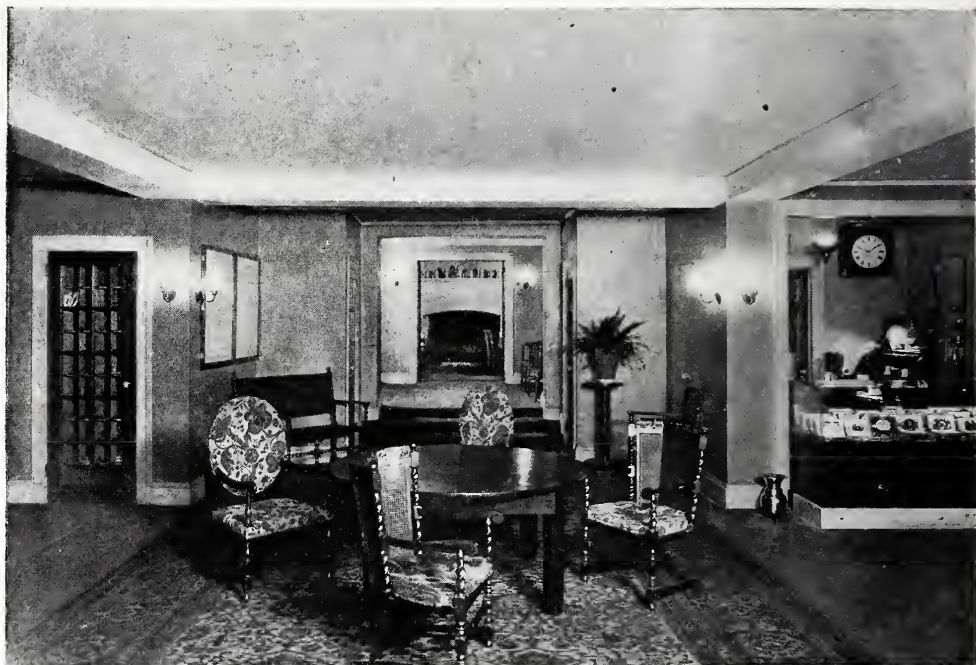
LOBBY—UNIVERSITY CLUB, SYRACUSE, N. Y. Taylor & Bonta, Architects.
