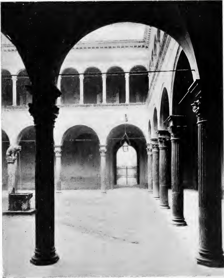
COURT OF BEVILACQUA PALACE, VERONA. TYPE OF THE RENAISSANCE ARCADED COURTYARD.
