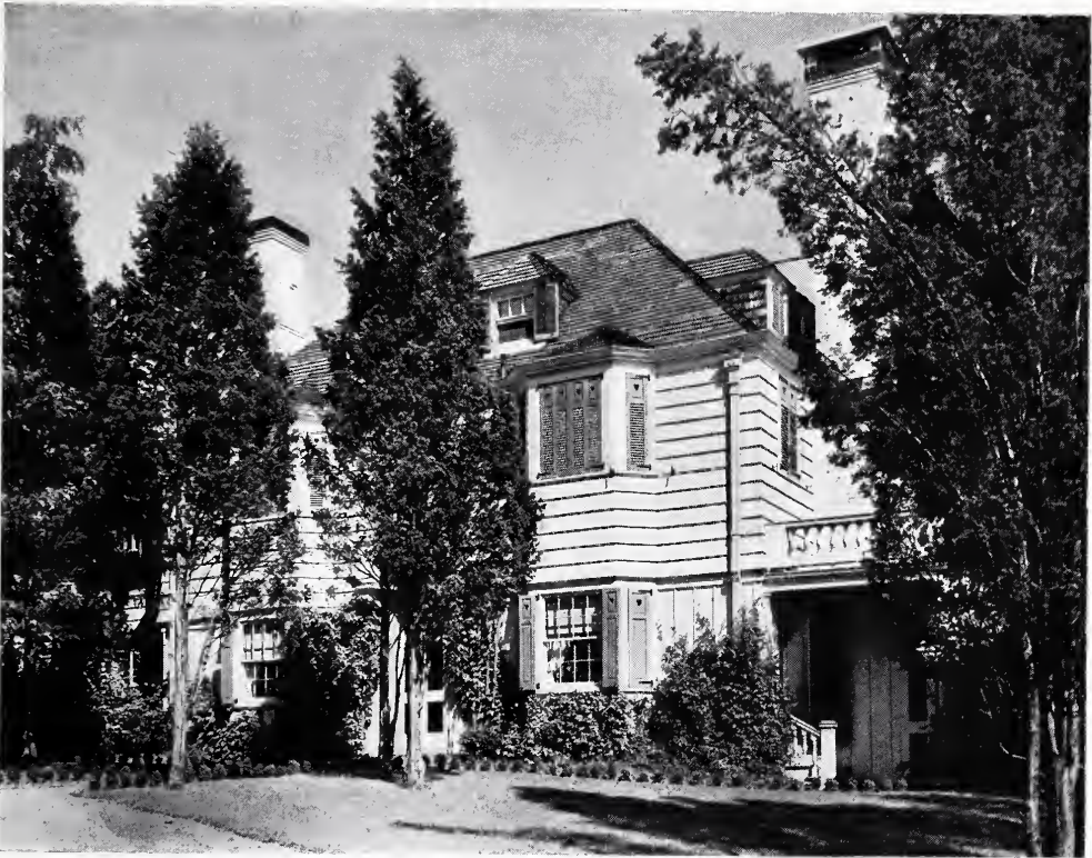
RESIDENCE OF DR. T. J. ABBOTT, CORNWALL-ON-HUDSON, N. Y. Parker Morse Hooper, Architect.
