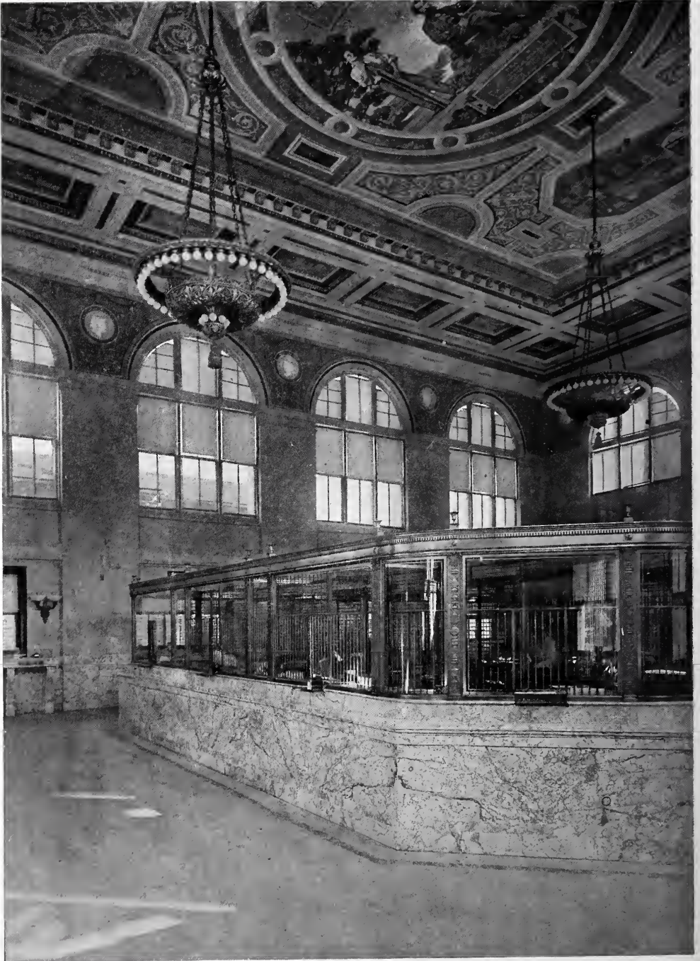
TITUSVILLE TRUST COMPANY'S BUILDING, TITUSVILLE, PA. ALFRED C. BOSSOM, ARCHITECT.
