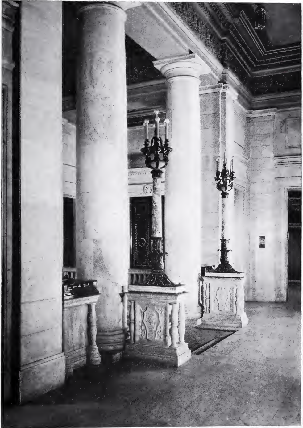
TRUST DEPARTMENT LOBBY AT HEAD OF STAIR FROM MAIN BANKING ROOM—GUARDIAN SAVINGS AND TRUST COMPANY'S BUILDING, CLEVELAND, OHIO. WALKER & WEEKS, ARCHITECTS.
