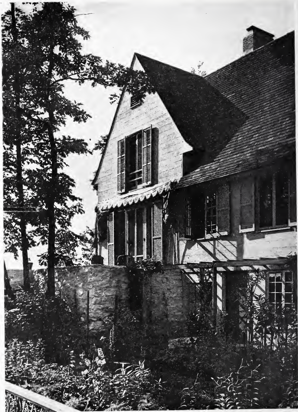
DETAIL—COTTAGE IN CONNECTICUT MURPHY & DANA, ARCHITECTS.
