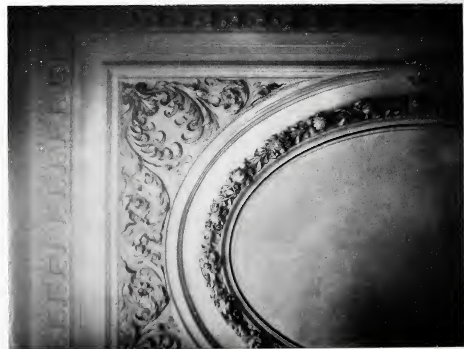
STAIRCASE CEILING—THE PYNES.
