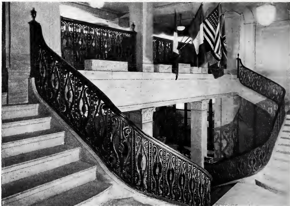
HOTEL CLEVELAND, CLEVELAND, OHIO. Graham, Anderson, Probst & White, Architects.
