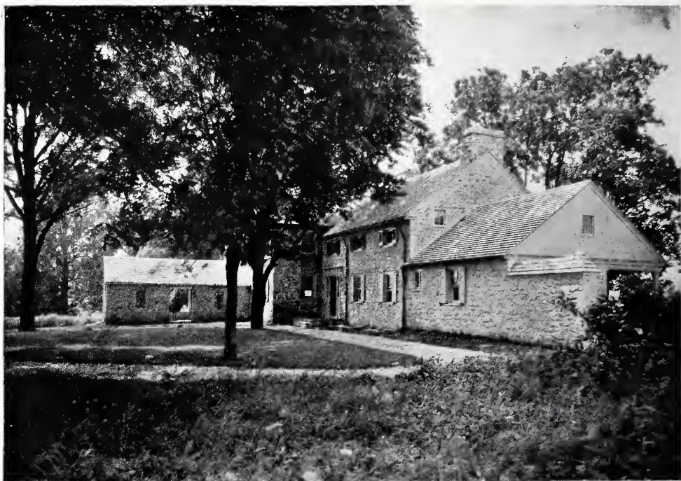
VIEW FROM NORTHEAST—RESIDENCE OF ELLIS Y. BROWN, JR., ESQ., DOWNINGTOWN, PA. Mellor & Meigs, Architects.
