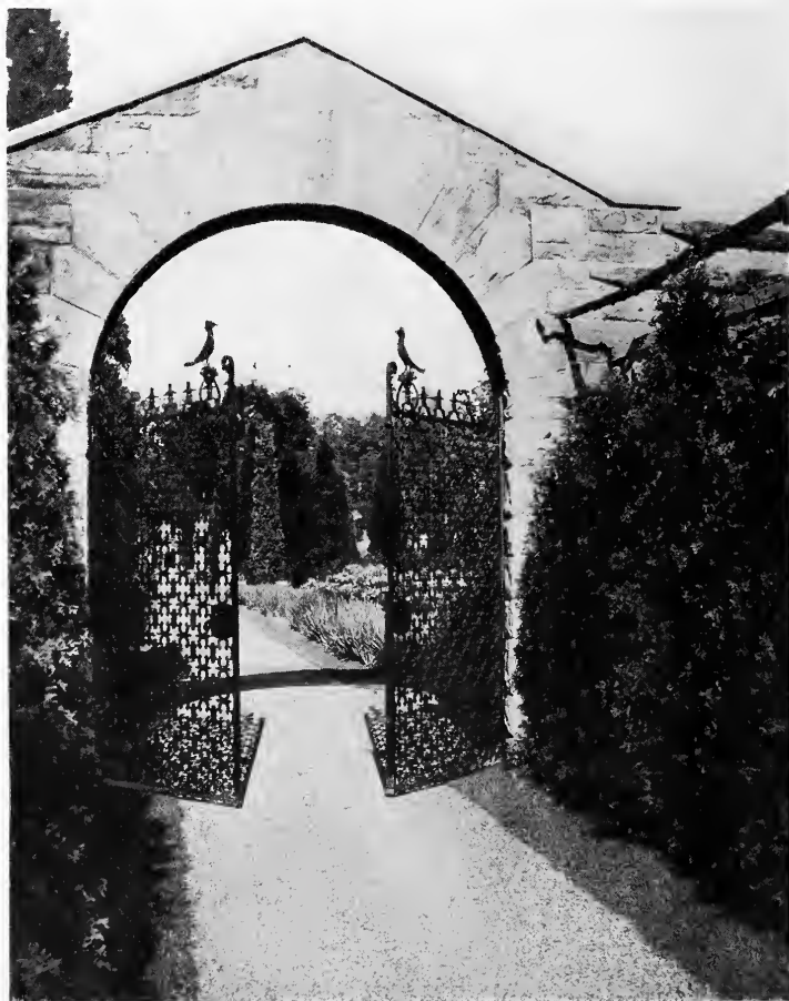
BLUE JAY GATE, OR THE VEHICLE ENTRANCE TO THE WHITE GARDEN. MASONRY OF NATIVE PATTON SANDSTONE IN WARM LIGHT-BROWN TINTS.
