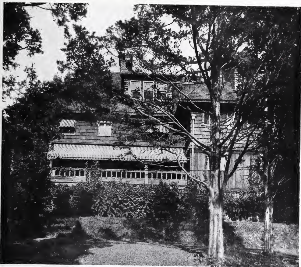
RESIDENCE OF LAWRENCE F. ABBOTT, ESQ., CORNWALL-ON-HUDSON, N. Y. Parker Morse Hooper, Architect.
