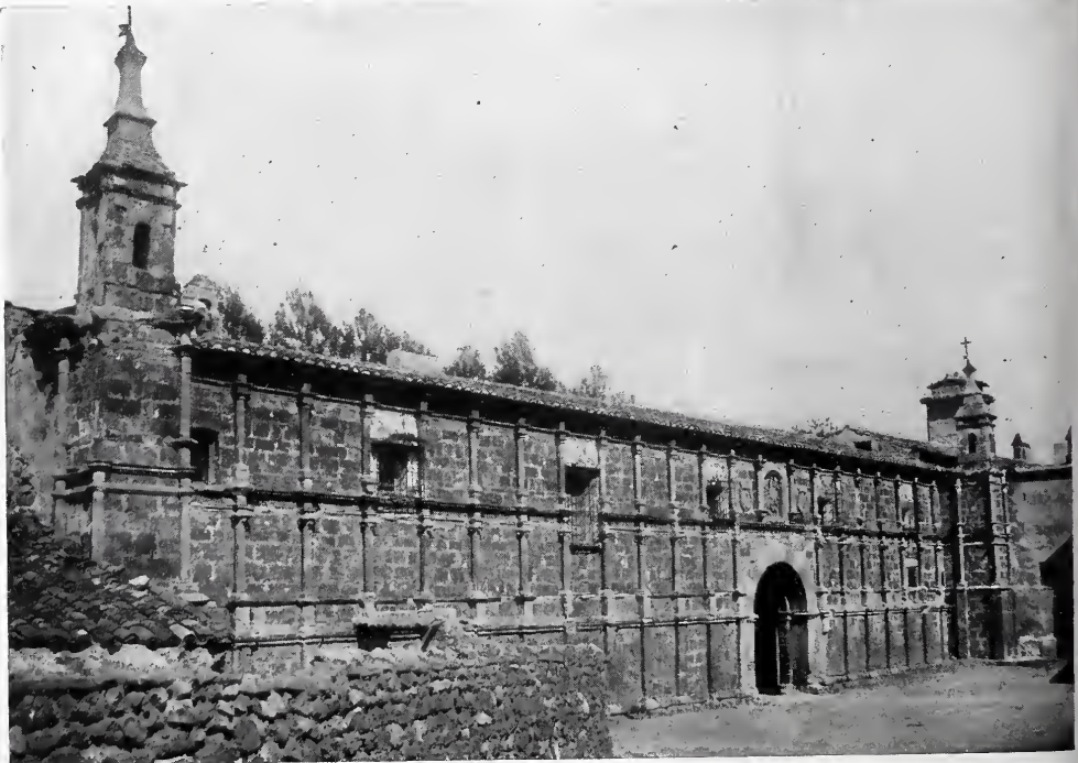
FAÇADE OF MONASTERY AT PIEDRA, SPAIN. ORDERS EMPLOYED FRANKLY AND OBVIOUSLY AS A WALL DECORATION.
