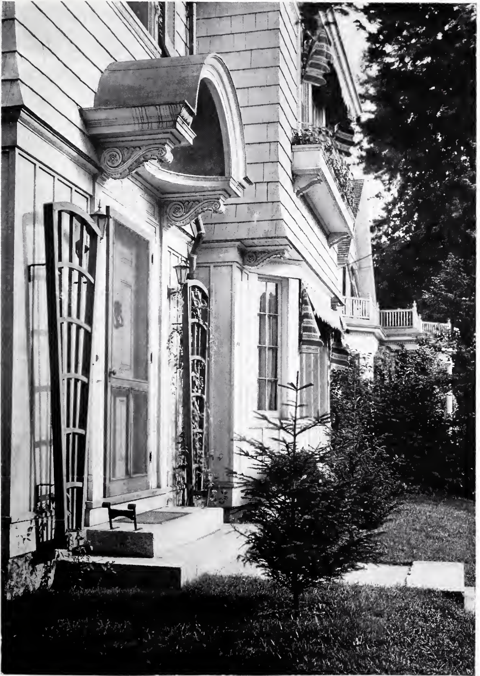
RESIDENCE OF DR. EDMUND F. CURRY, FALL RIVER, MASS. PARKER MORSE HOOPER, ARCHITECT.
