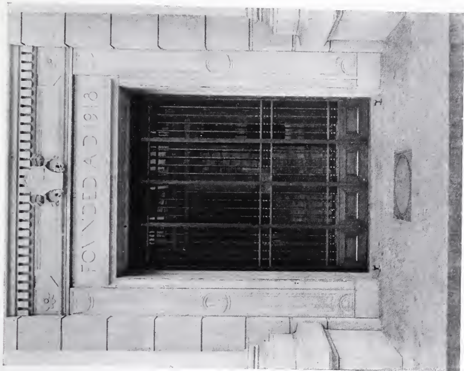
TITUSVILLE TRUST COMPANY'S BUILDING, TITUSVILLE, PA. Alfred C. Bossom, Architect.
