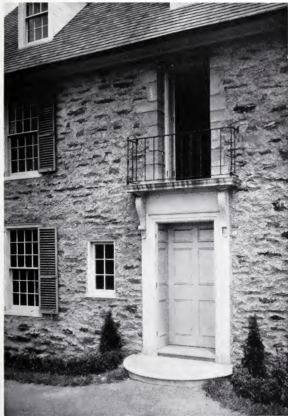
ENTRANCE DETAIL—TWO HOUSES FOR THE MORRIS ESTATE, OVERBROOK, PHILADELPHIA. MELLOR, MEIGS & HOWE, ARCHITECTS.
