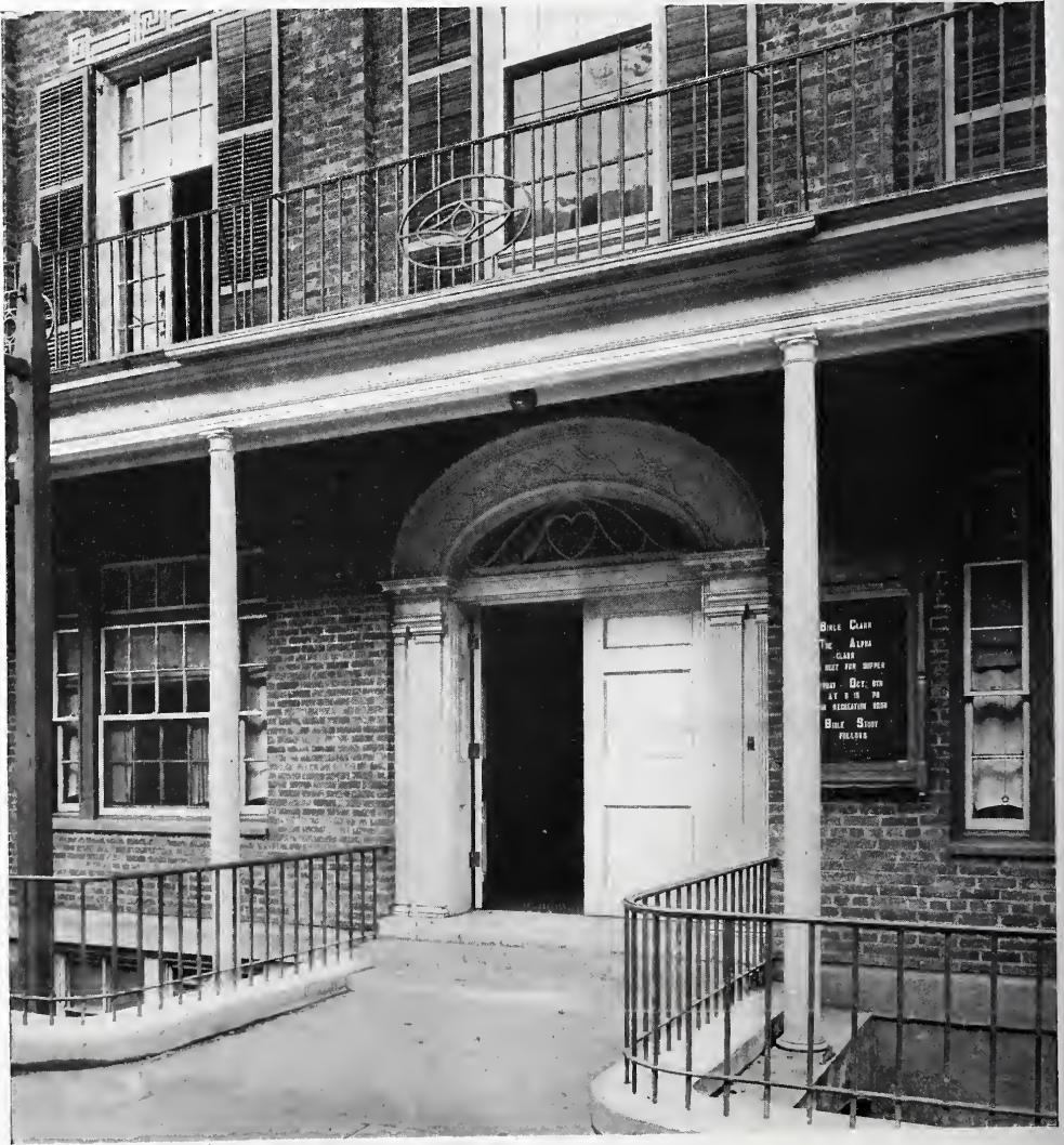
ENTRANCE TO ADMINISTRATION SIDE —Y. W. C. A. BUILDING, SYRACUSE, N. Y. TAYLOR & BONTA, ARCHITECTS.
