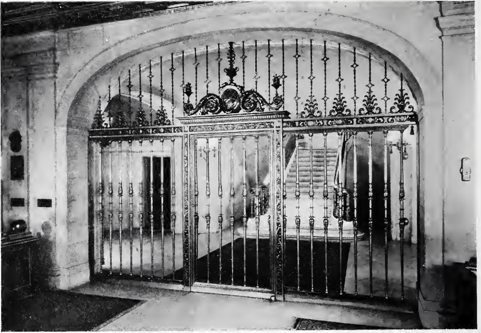
GRILLE OF SAFE DEPOSIT DEPARTMENT—GUARDIAN SAVINGS AND TRUST COMPANY'S BUILDING, CLEVELAND, OHIO. Walker & Weeks, Architects.
