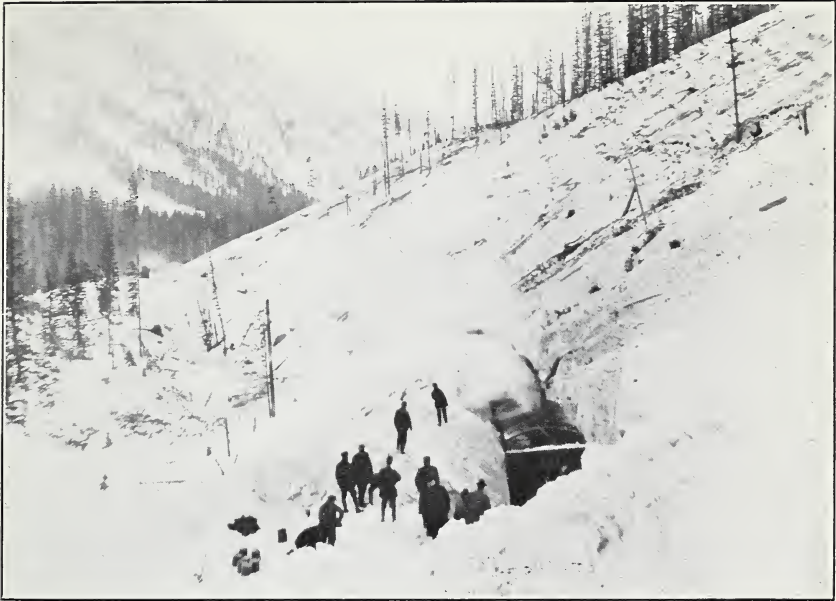
FIG. 1.—CLEARING SNOW AND DÉBRIS FROM THE RAILROAD TRACKS AFTER THE BERNE SLIDE, WHICH CAME FROM THE DEFORESTED HILLSIDE ON THE RIGHT AND COVERED THE TRACK FOR A THIRD OF A MILE.
