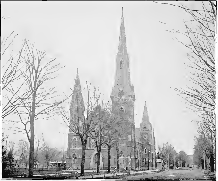
Church Building of today, dedicated 1879
