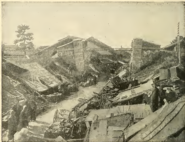
FIG. 246. Effect of earthquake in Japan, 1891.
