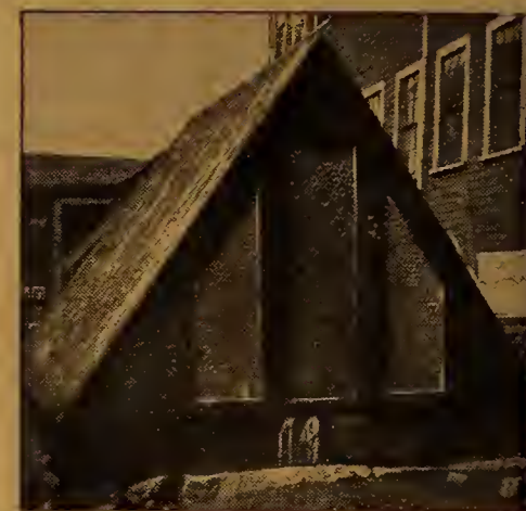
An A-shaped brooder coop or laying house covered entirely with prepared roofing except the open wire-covered front. Easy to build any size desired.
