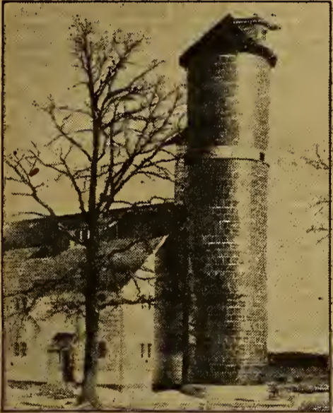
Combination tile silo and water tank
