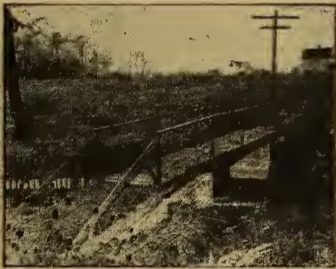
The substantial concrete work makes this bridge safe at all times
