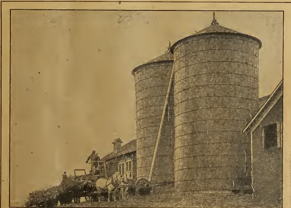
Two silos of average capacity give better results than one huge one. These are wood-stave silos on concrete foundations
