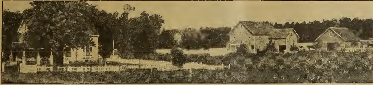
These buildings of an Iowa hog farm are all painted gray with white trimmings, ready-mixed paint being used. Two coats were applied in 1907, one coat in 1911, and one coat in 1915
