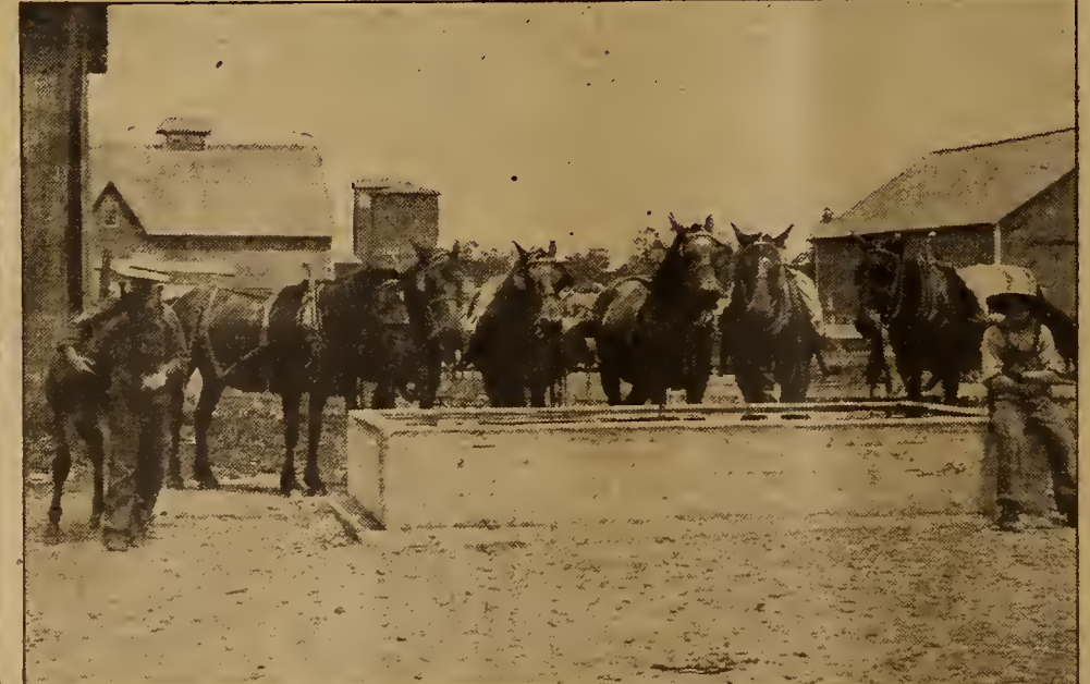
Here is a concrete water trough that has proved to be a very satisfactory improvement on this Middle West farm
