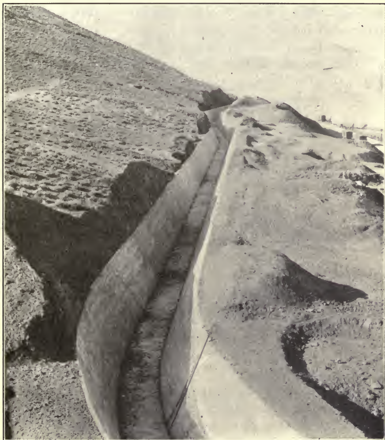
FIG. 23.—Concrete Lining, Truckee-Carson Canal, Nevada.
