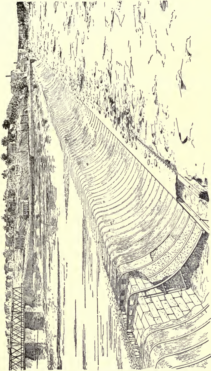
PLATE VIII.—Iron-faced Rollerway Weir, Cohoes, N. Y.
