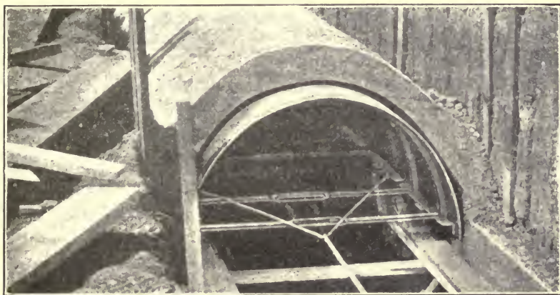
FIG. 131.—Travelling Forms for Moulding Concrete Pipe.
