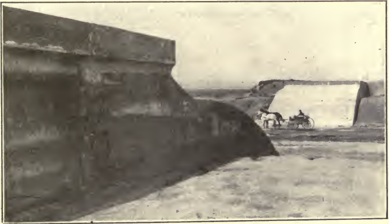
PLATE XIX B.—Siphon Crossing Under Rawhide Creek, Interstate Canal, Nebraska-Wyoming.
