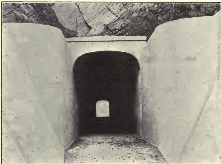
FIG. 18.—Tunnel Portal and Lining Truckee-Carson Canal, Nevada.
