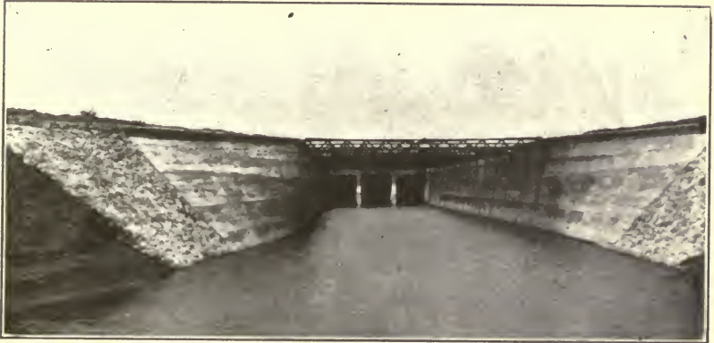
PLATE XIX A.—Inlet to Rawhide Siphon, Interstate Canal, Nebraska-Wyoming.
