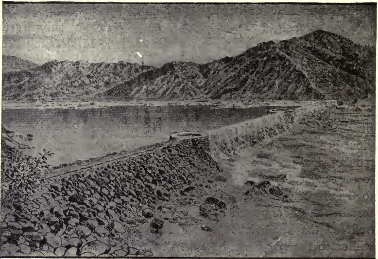
FIG. 159.—View of San Fernando Submerged Dam.
