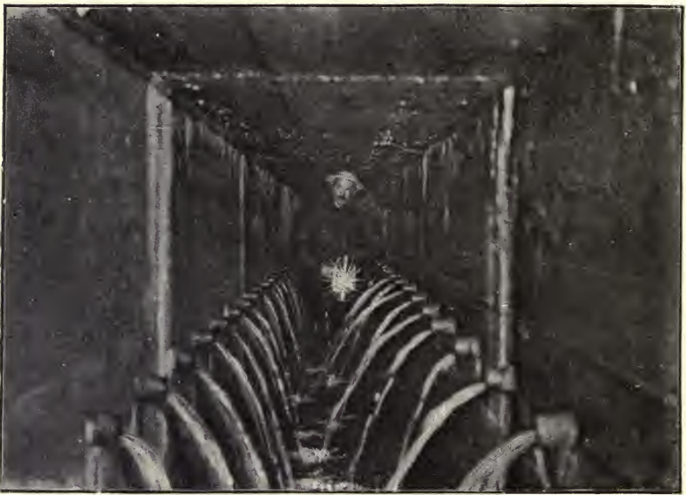
FIG. 13.—Subterranean Water Tunnel and Feed-wells, California.
