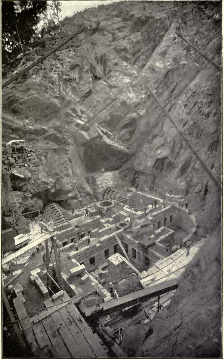
PLATE XXIV.—Excavating Foundation for New Croton Dam and Gate-house.
