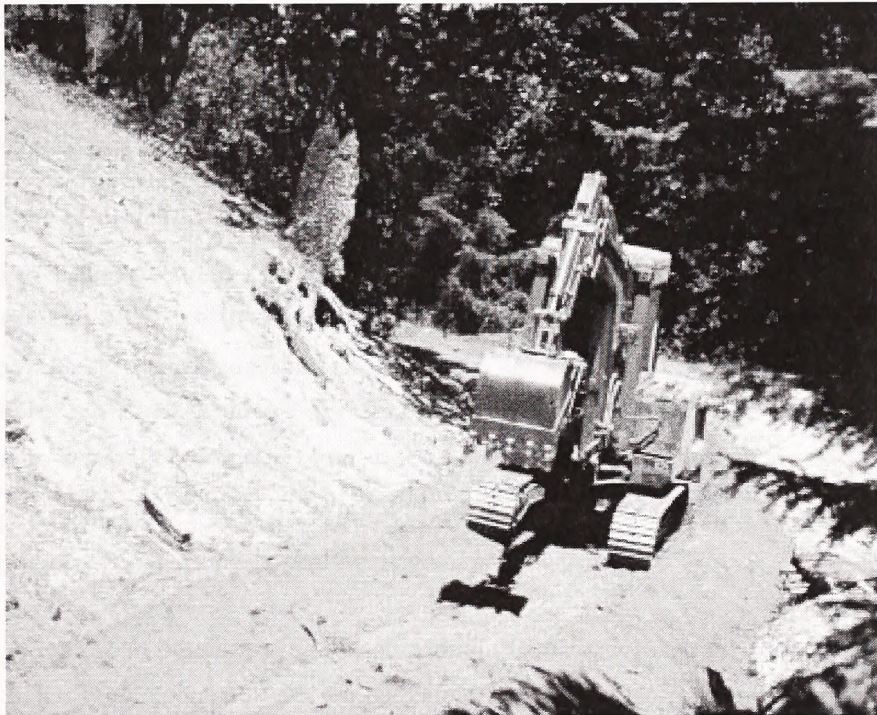
Road decommissioning requires the use of heavy equipment.
