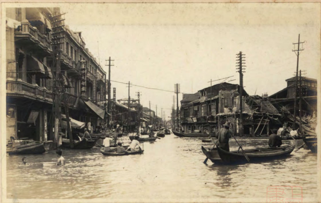
The Collapsed Hotel at Taichemen. 大智門倒塌之迎賓旅館
