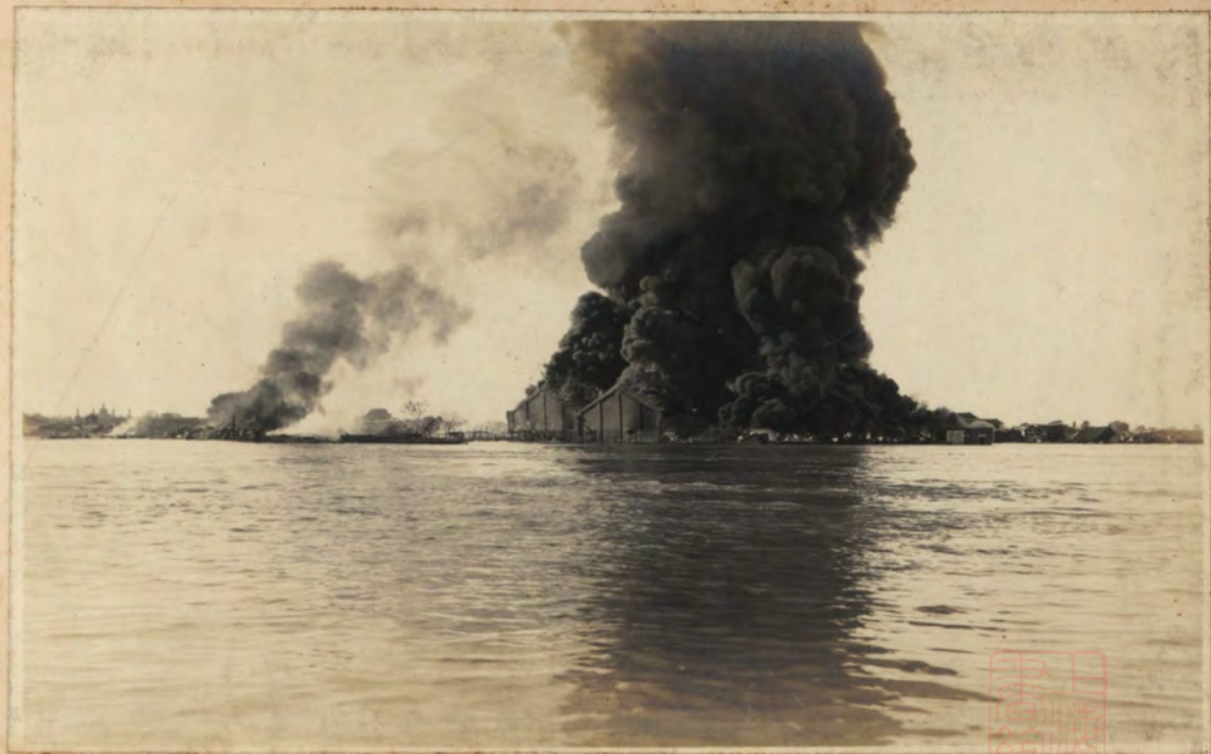
The Fire at The Texas Co. Installation, Aug. 27th. 1931 被燒之德士古油棧
