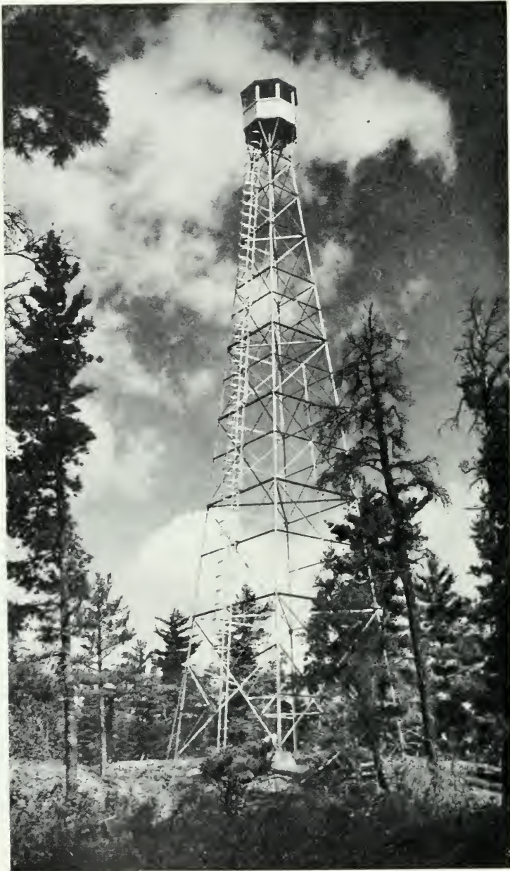
FIRE DETECTION TOWER IN KENORA DISTRICT. FROM SUCH TOWERS AS THIS, FIRES MAY BE QUICKLY DETECTED, AND BY USE OF TELEPHONE OR RADIO, THE FIRE-FIGHTING CREWS MAY BE NOTIFIED IMMEDIATELY
