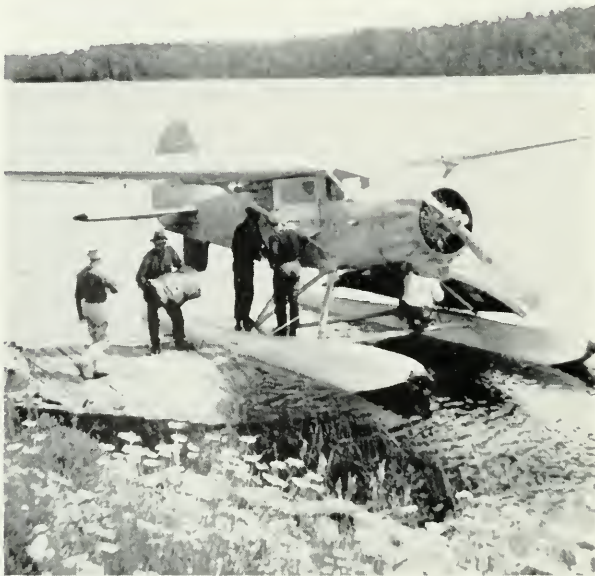
PLANE BEING USED TO TRANSPORT CONSTRUCTION MATERIALS TO NORTHERN OUTPOST
