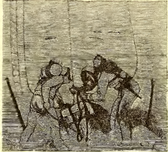
DIVERS AT WORK UNDER WATER.
