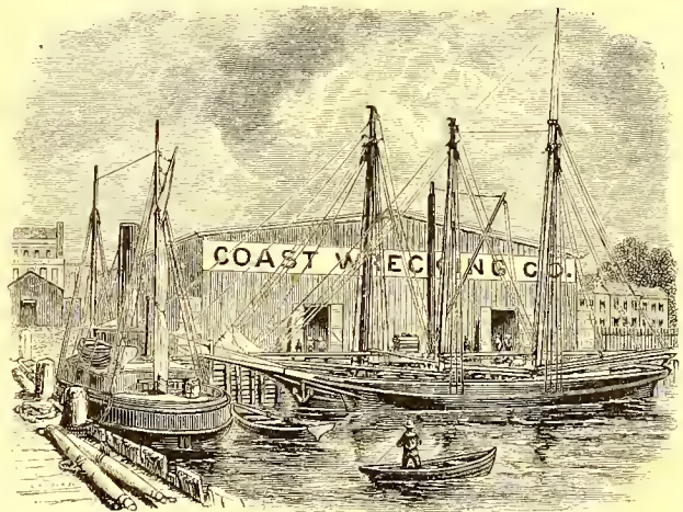
COAST-WRECKERS' STATION ON STATEN ISLAND.
