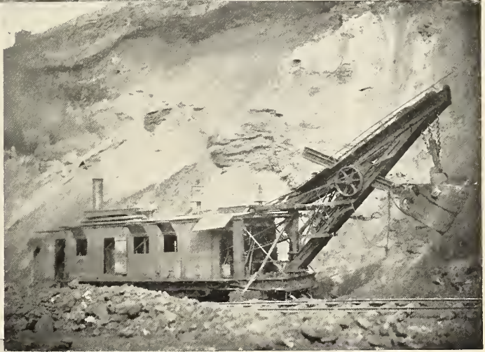
FIG. 3. STEAM SHOVEL SCOOPING UP ORE.
