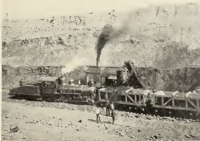
FIG. 4. STEAM-SHOVEL MINING AND LOADING CARS AT ONE OPERATION.
