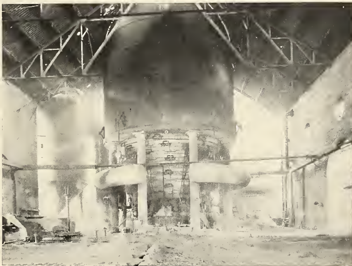
FIG. 10. INTERIOR OF THE CASTING-HOUSE, SHOWING THE LOWER PART OF A BLAST-FURNACE.
