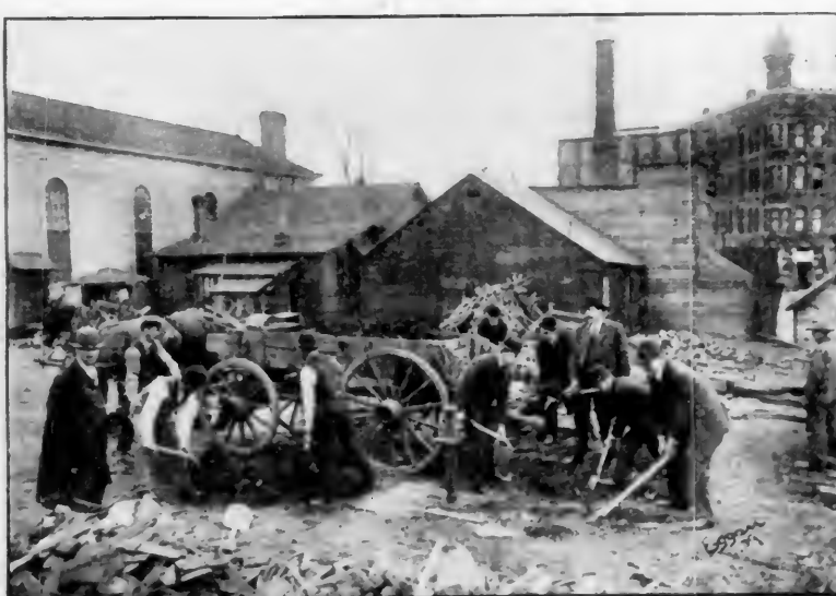
The above photograph represents the breaking of ground for the new Southern Theatre, located at Cedar and Washington Avenues, Minneapolis, Minnesota, this ceremony having taken place on May 12. This theatre will be completed by August 20, this year and will be fire-proof throughout, with a stage 22x22, the building being 50x125 and having a capacity of about 850. The cost will be about $50,000. Four shows per day of vaudeville at a ten cent straight price of admission will be the nature of the entertainment offered. The theatre is being built by the Southern Amusement Company and will be managed by Mr. W. A. Kelly.
